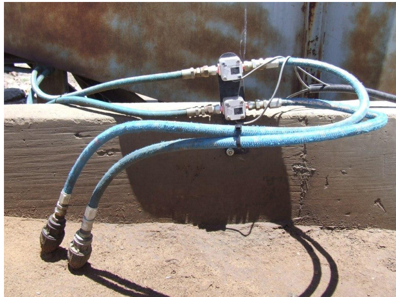
Figure 11: Installation of fuel flow metres.
