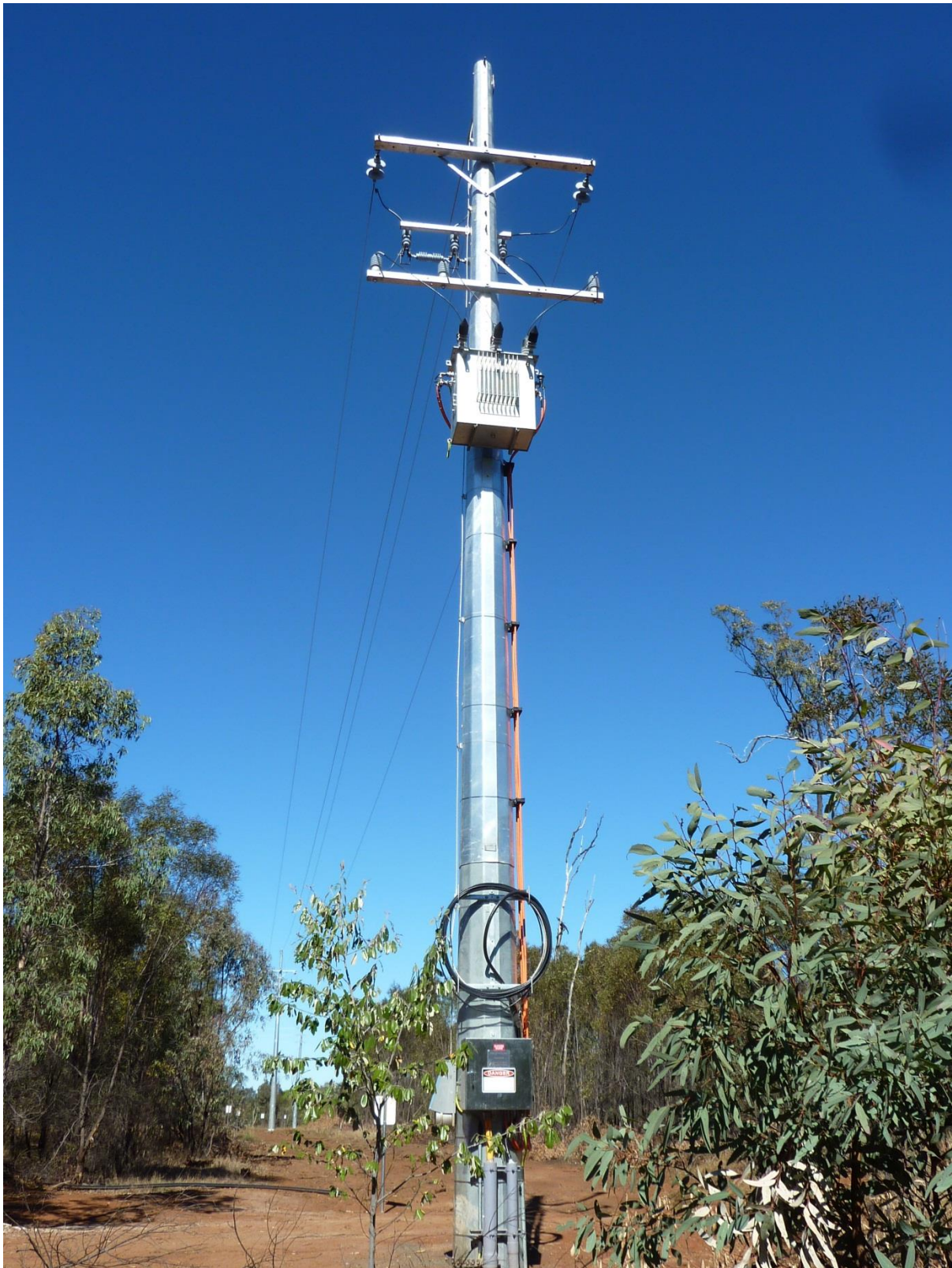
Figure 4.8 – Typical 11kV/415V pole top transformer installation
