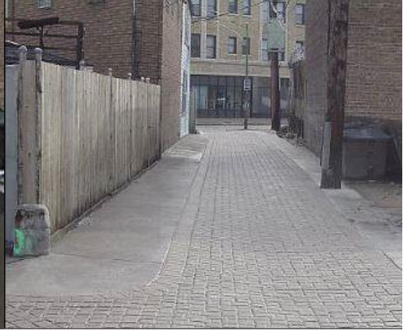
Figure 4.9 - The same alley after conversion into a 'Green Alley' (Chicago Department of Transportation 2010).
