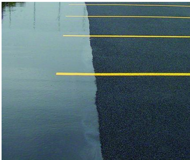
Figure 3.1 - Comparison of appearance of conventional asphalt (left) & porous asphalt (right) (National Asphalt Pavement Association n.d.)
