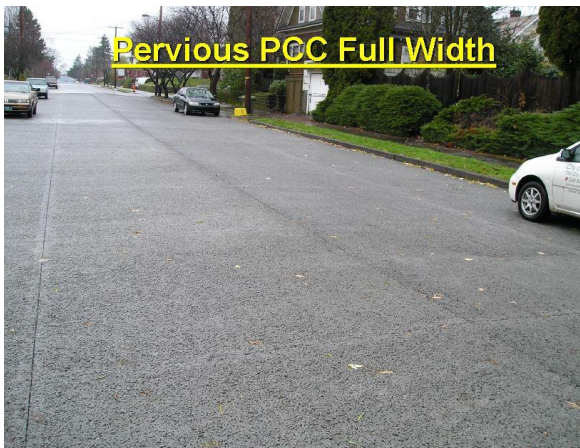
Figure 10.3 - Completed full-width PC street
