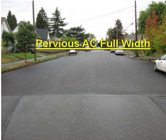
Figure 10.1 - Completed full-width PA street
