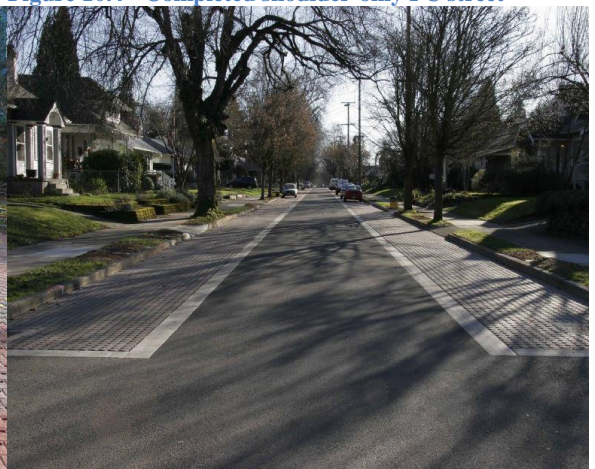
Figure 10.6 - Completed shoulder-only PP street
