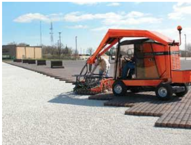
Figure 3.12 - This machine provides a mechanical means of laying blocks of pavers (Interlocking Concrete Pavement Institute 2008).
