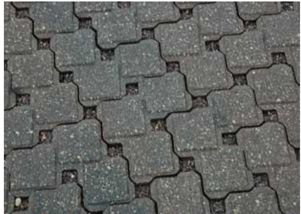
Figure 3.9 - Permeable interlocking concrete pavers (PICP) (Landscape Online 2013)
