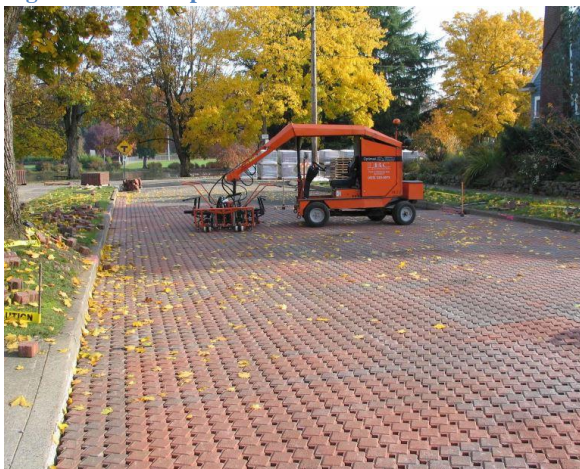
Figure 10.5 - Completed full-width PP street
