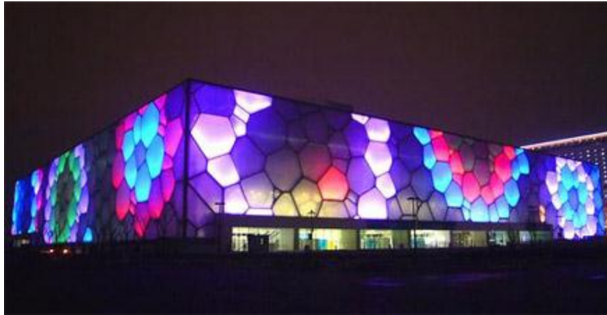
Figure 5.9: Beijing National Aquatics Stadium at night showcasing its ability to produce many luminous colours in the ETFE bubbles (Architect 2008)
