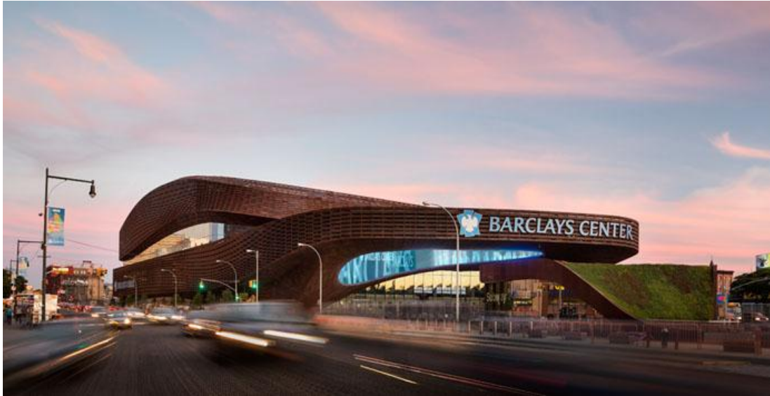
Figure 5.12: The Barclays Center in Brooklyn, New York. View of the main plaza with the 'Oculus' and the subway station in the foreground (AECOM 2013)
