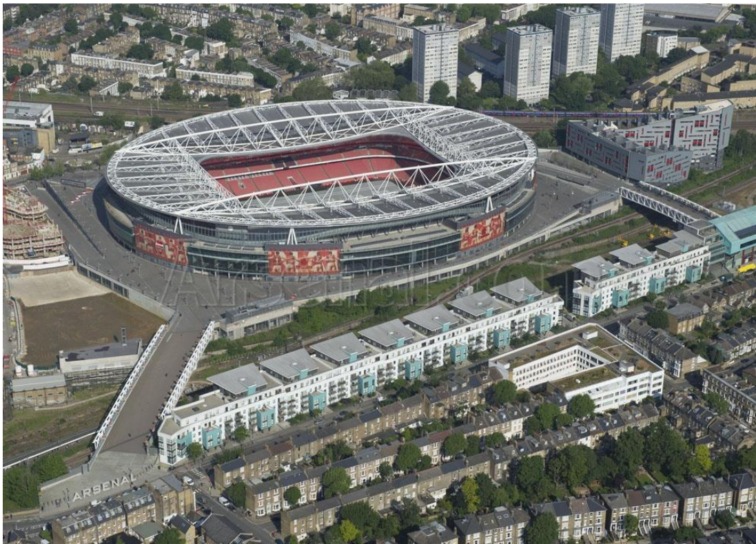
Figure 4.5: Emirates Stadium and surrounds in North London, England (Arsenal Football Club 2013)
