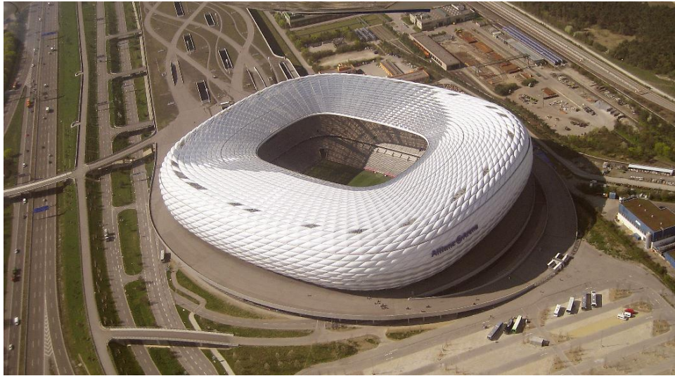
Figure 5.11: Aerial view of Allianz Arena (Allianz 2013)
