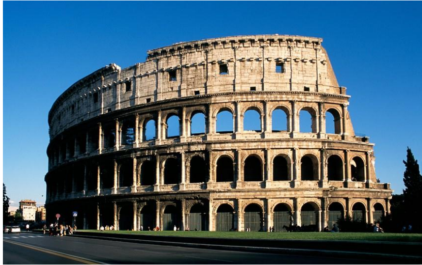
Figure 3.6: Exterior of the Colosseum in Rome, Italy illustrating the arches used for support (Squires 2012)
