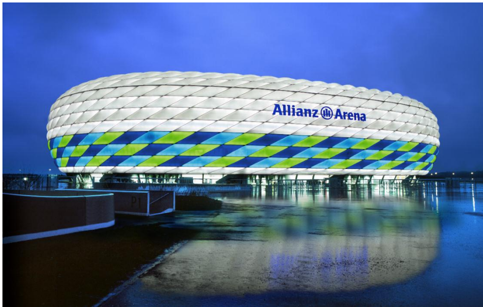
Figure 5.10: Allianz Arena in Munich, Germany with a number of its panels lit up with colour-changing LED lighting (Allianz Insurance 2013)
