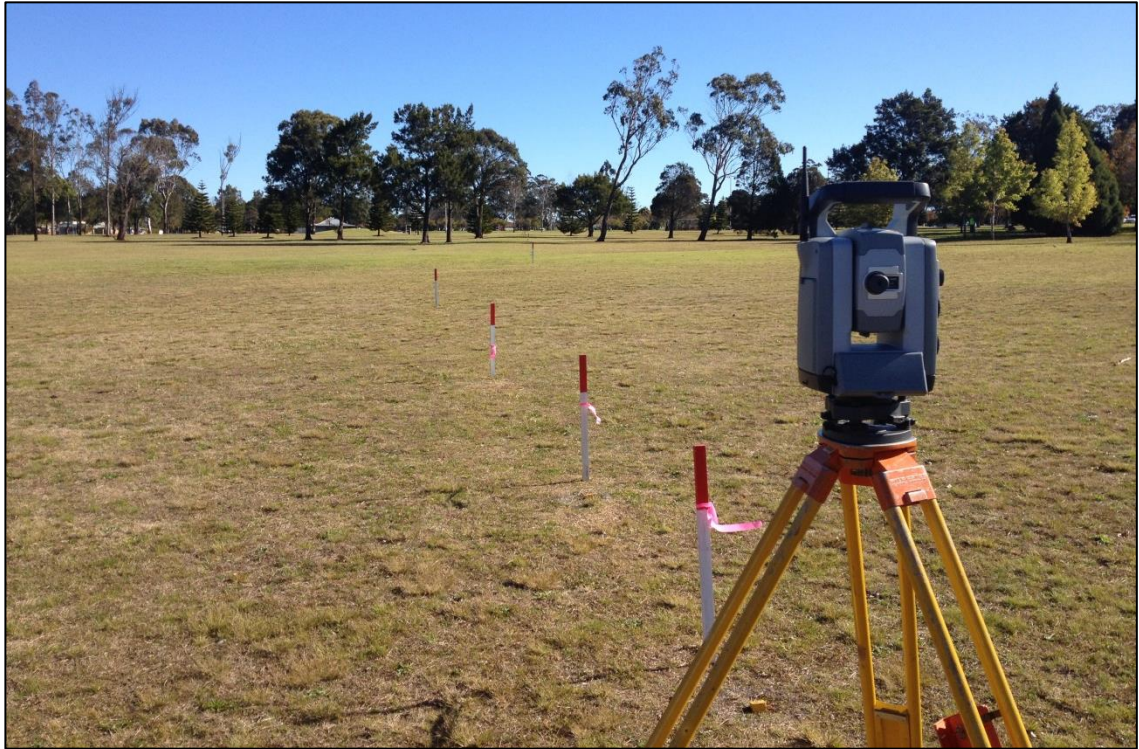
Figure 3.7 – Picture of the control array with the reference marks in the foreground and the BS and short line lengths going into the background
