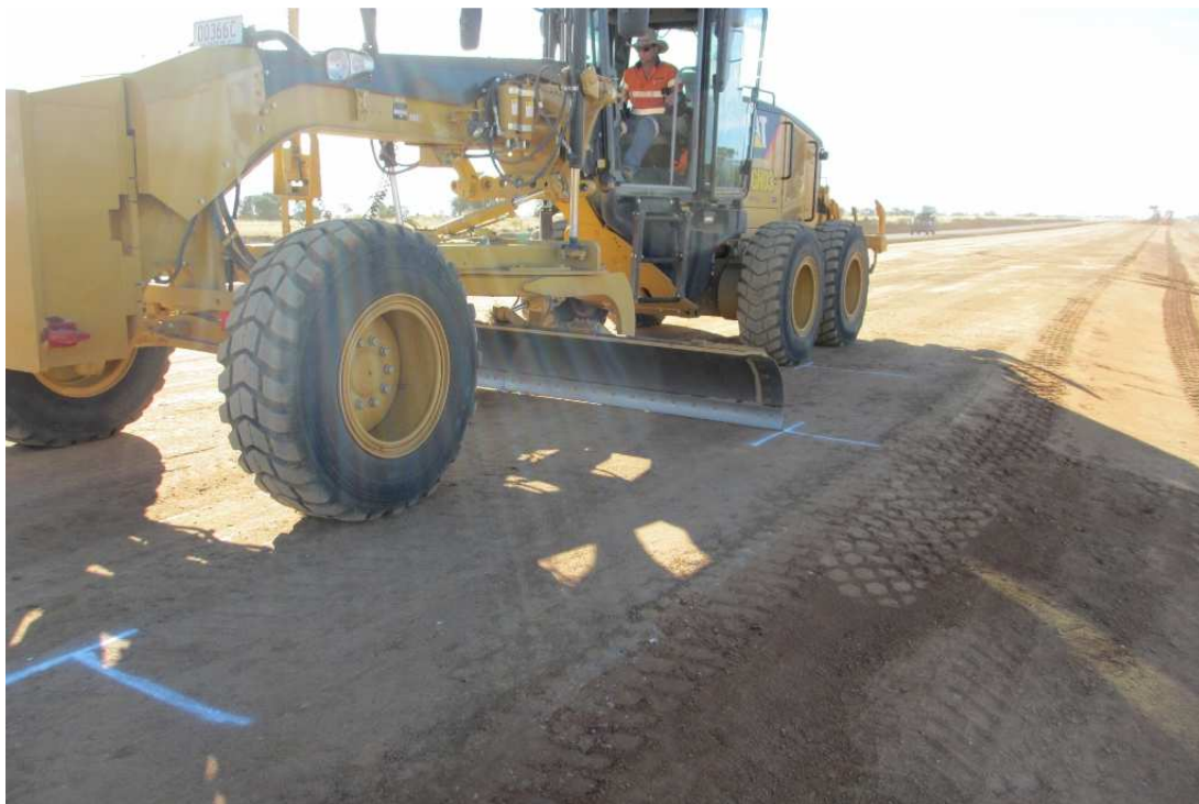
Figure 8-2 Trimble Guided Grader in Position 2 Landsborough Highway
