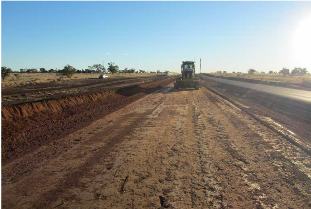
Figure 10-1 Field Test 1 Finished Surface Level
