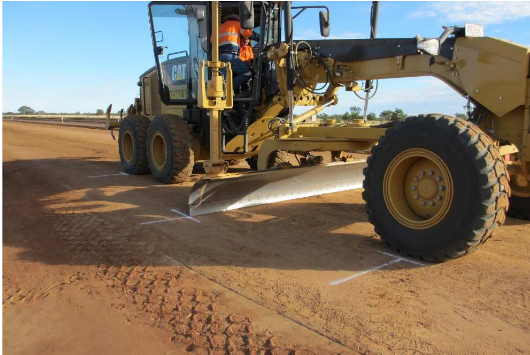
Figure 8-1 Trimble Guided Grader in Position 1 Landsborough Highway
