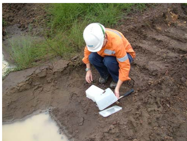
Flocculant block is removed from packaging
