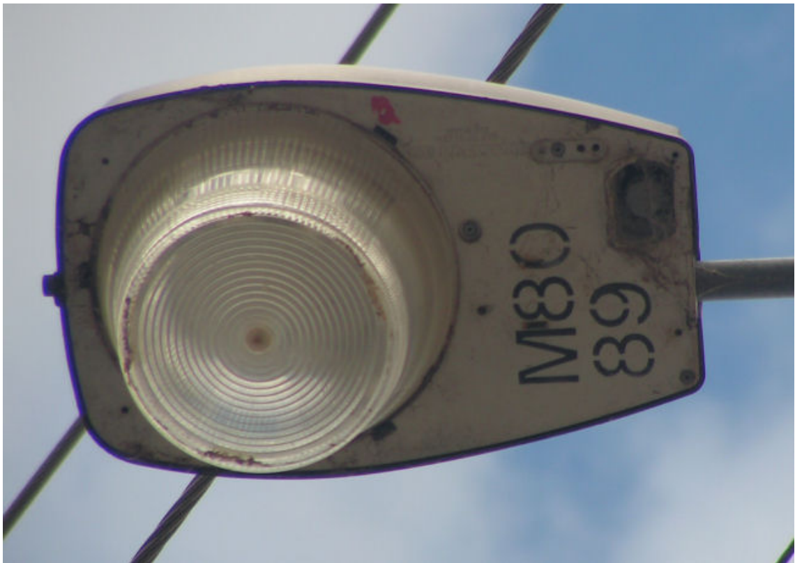
Figure 3-9 Existing Sylvania 80W MV luminaire manufactured in 1989
