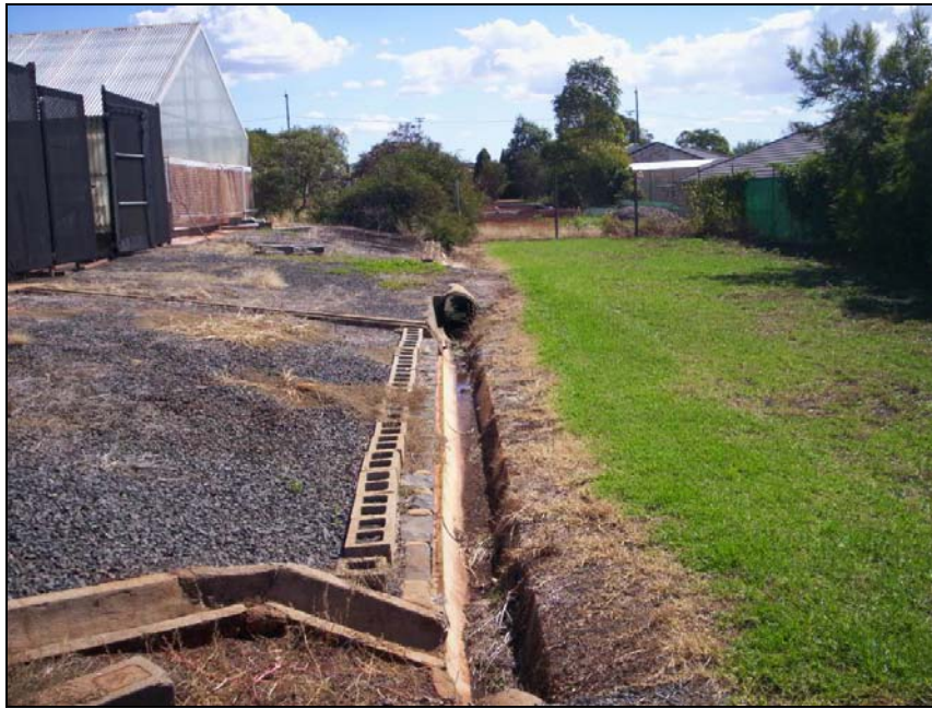
Figure C1a – Overlooking Drainage infrastructure towards potential harvest area
