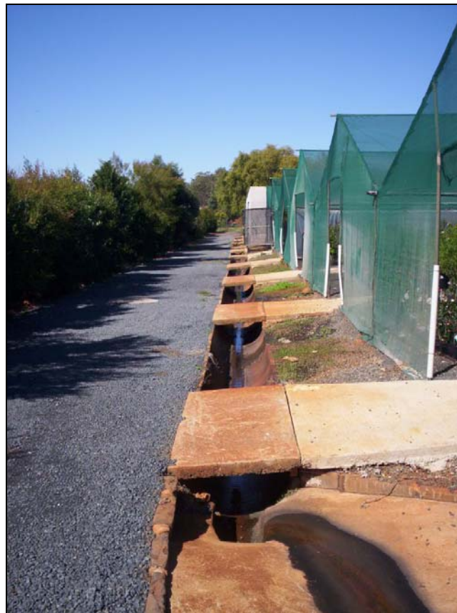
Figure C1b – Looking east along spoon drain
