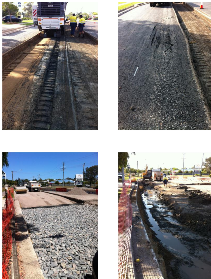
Figure 57: Buderim St, Currimundi - Construction Photos Subgrade Replacement
