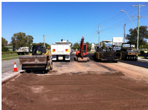
Figure 56: Buderim St, Currimundi - Construction Photos of Unsuitable Subgrade Locations
