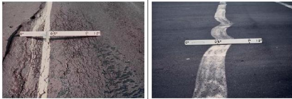
Figure 15: Typical Shoving Defect (Austroads, 2009)
