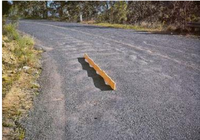
Figure 13: Defect Type: Corrugations (Austroads, 2009)
