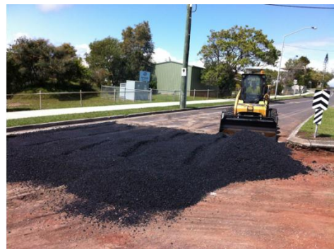
Figure 56: Buderim St, Currimundi - Construction Photos of Unsuitable Subgrade Locations
