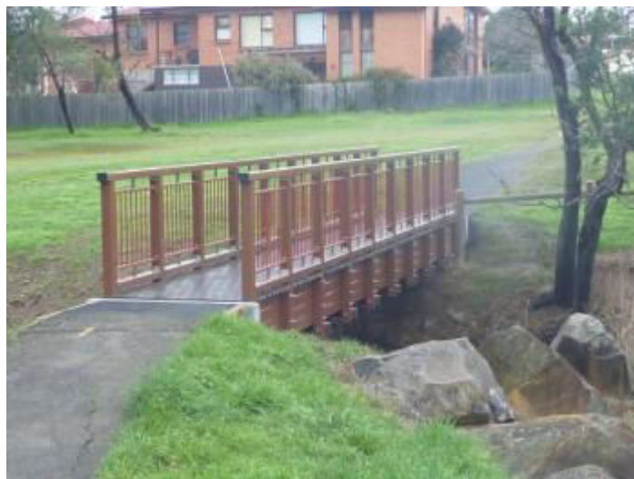
Figure 1.1: Composite fibre bridge in Tasmania, Australia
