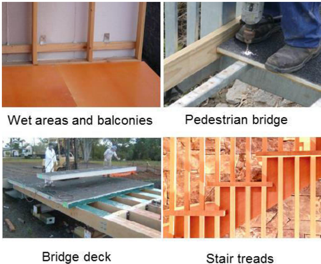
Figure 2.4: Structural Applications of Sandwich Panels
