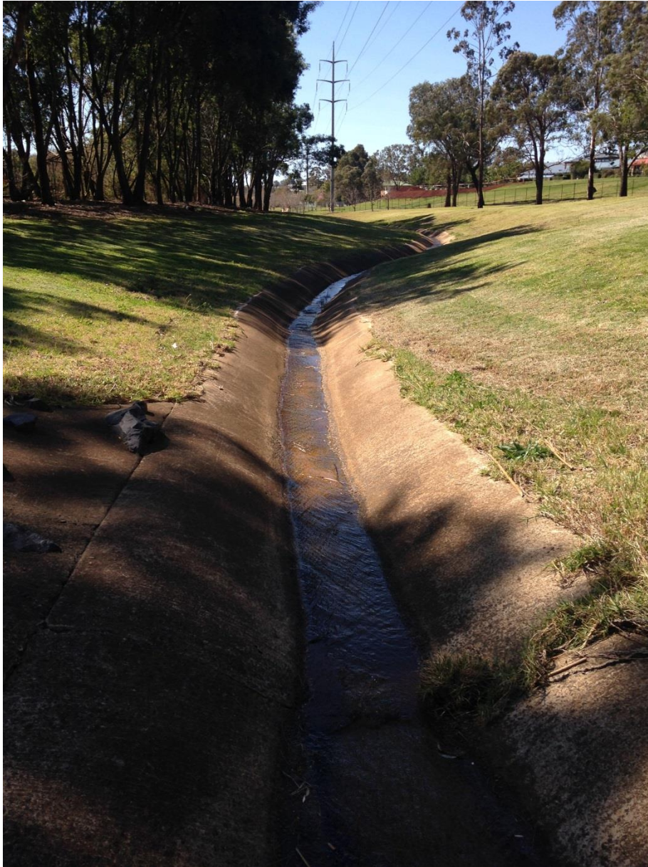
Figure 6: Concrete lining on the lowest part of West Creek in between Spring Street and Stenner Street in South Toowoomba as of August 2104.
