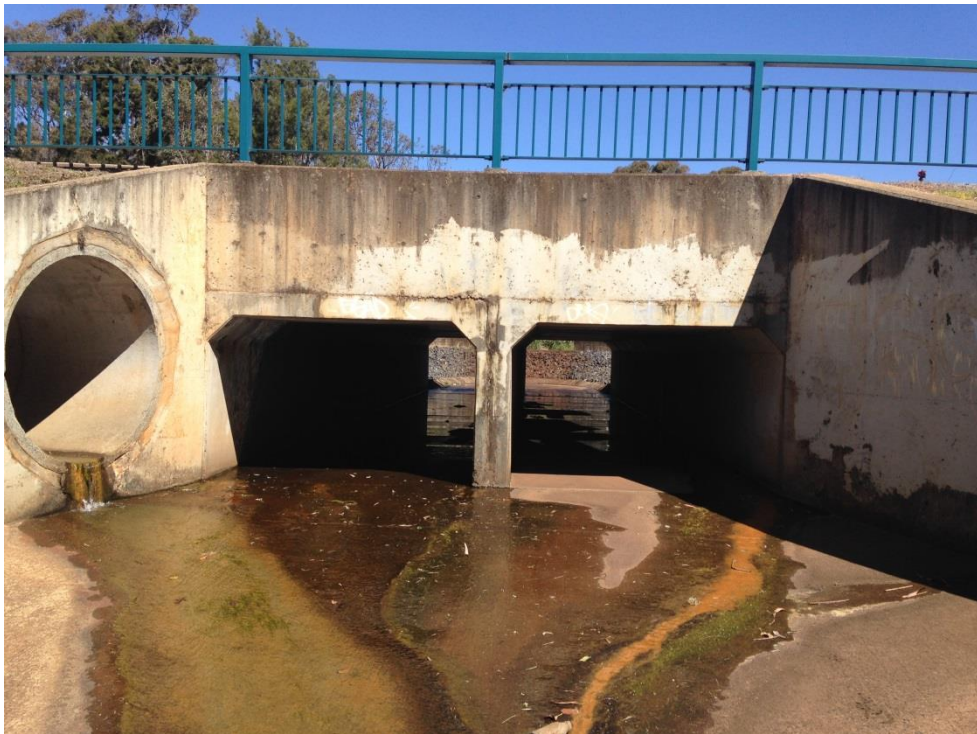
Figure 39: The piped drainage system used under the Spring Street road crossing funnelling the water in and out again taken in August 2014.
