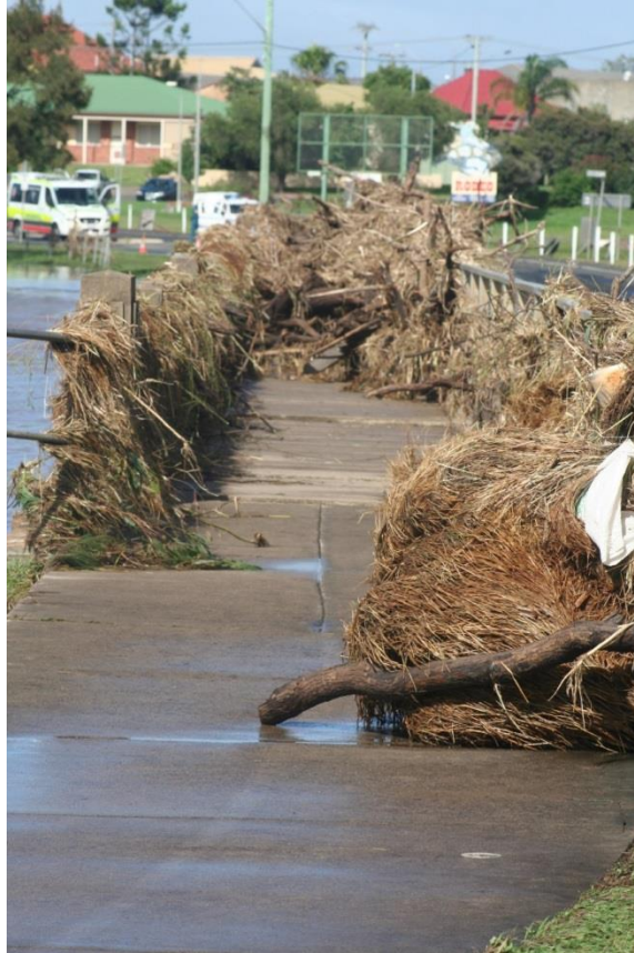
Figure 2.9 - Debris blockage on the O.O. Madsen after the 2011 floods (Warwick Daily News, 2011)
