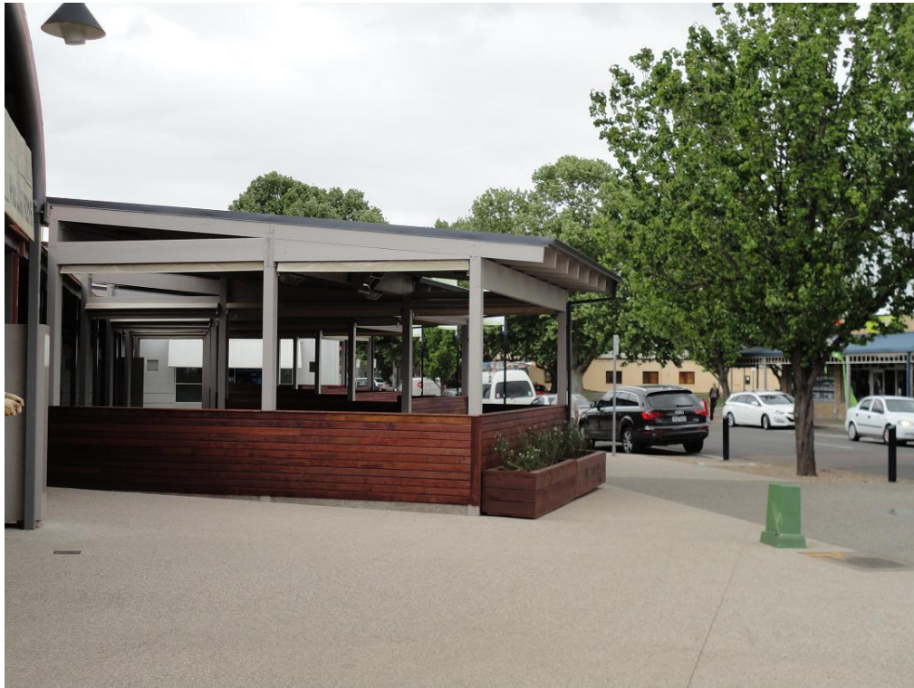
Figure 5.3 – the alfresco outdoor dining constructed in 2014. The proposed site and RSL building can be seen in the background.
