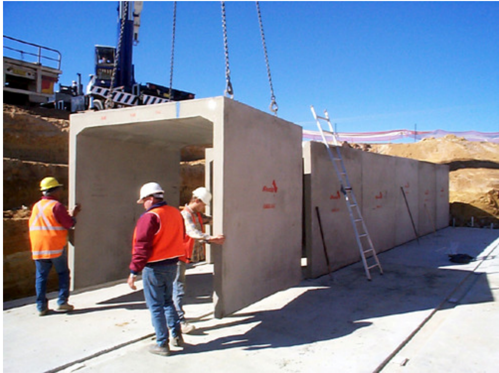
Figure 2-2 - Three-sided box culvert (Rocla 2014)
