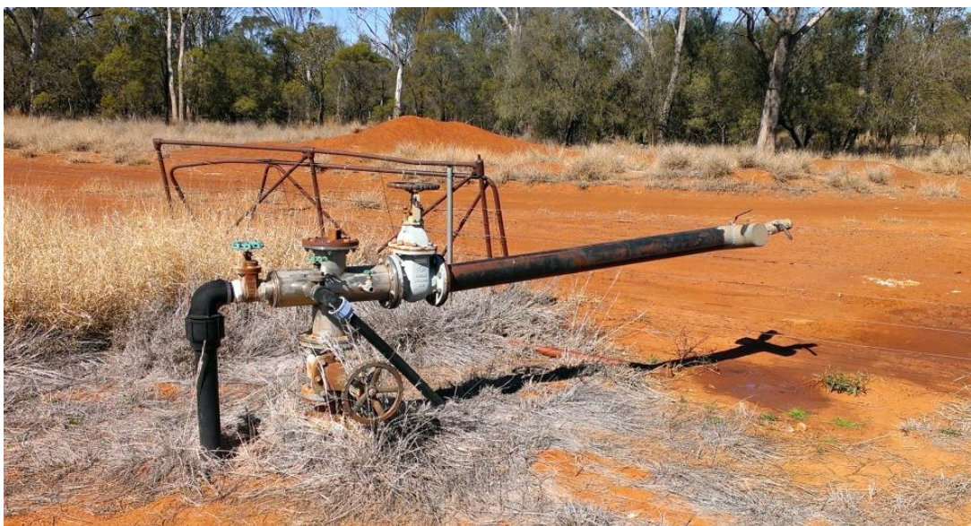
Figure 5.2. Bore head at "Tabooba" and typical ground conditions
