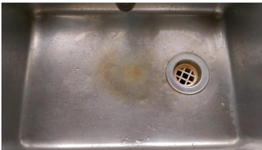
Figure 7.4. Staining on a sink at "Tabooba" due to water with a high mineral content
