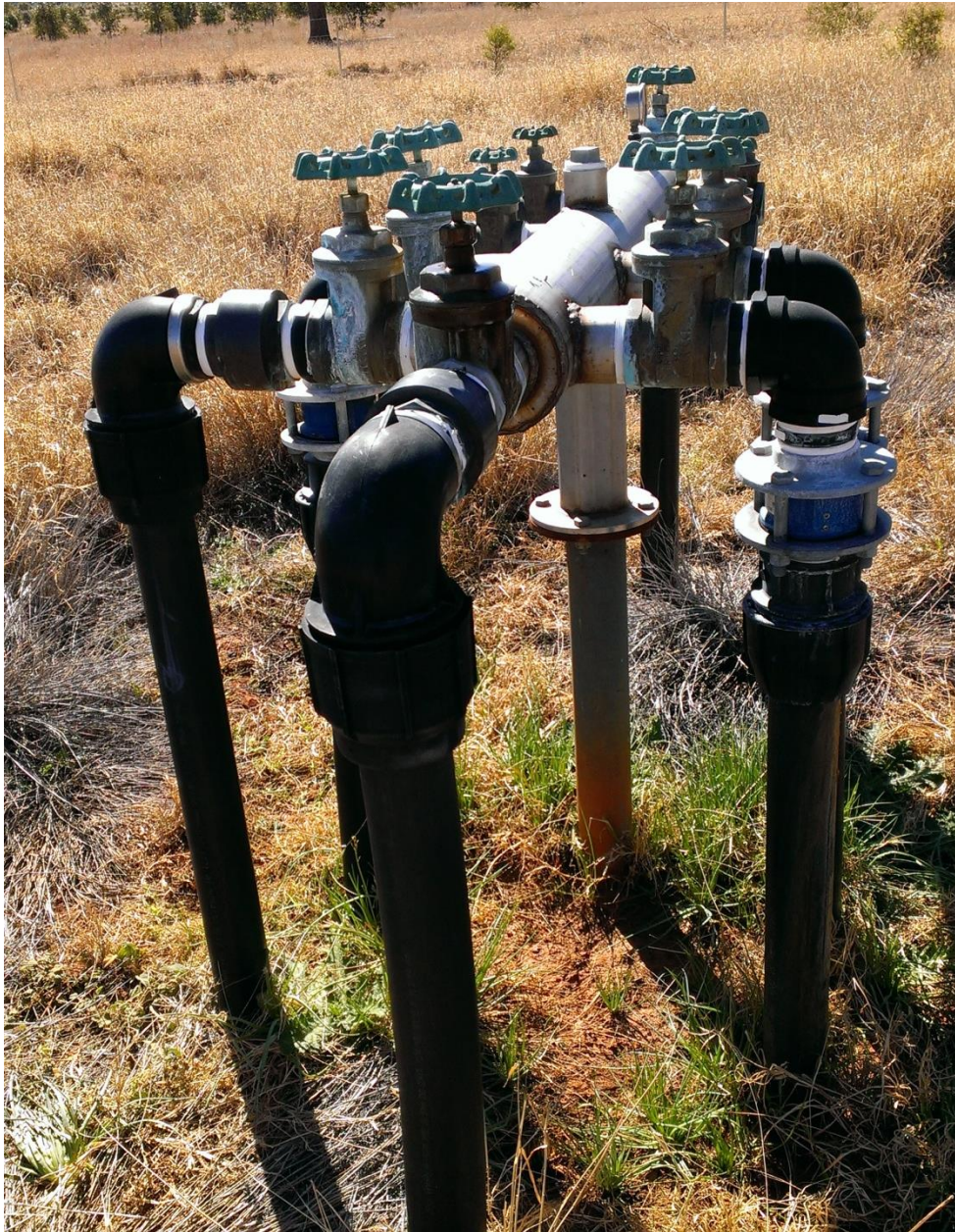
Figure 4.2. "Tabooba" distribution manifold
