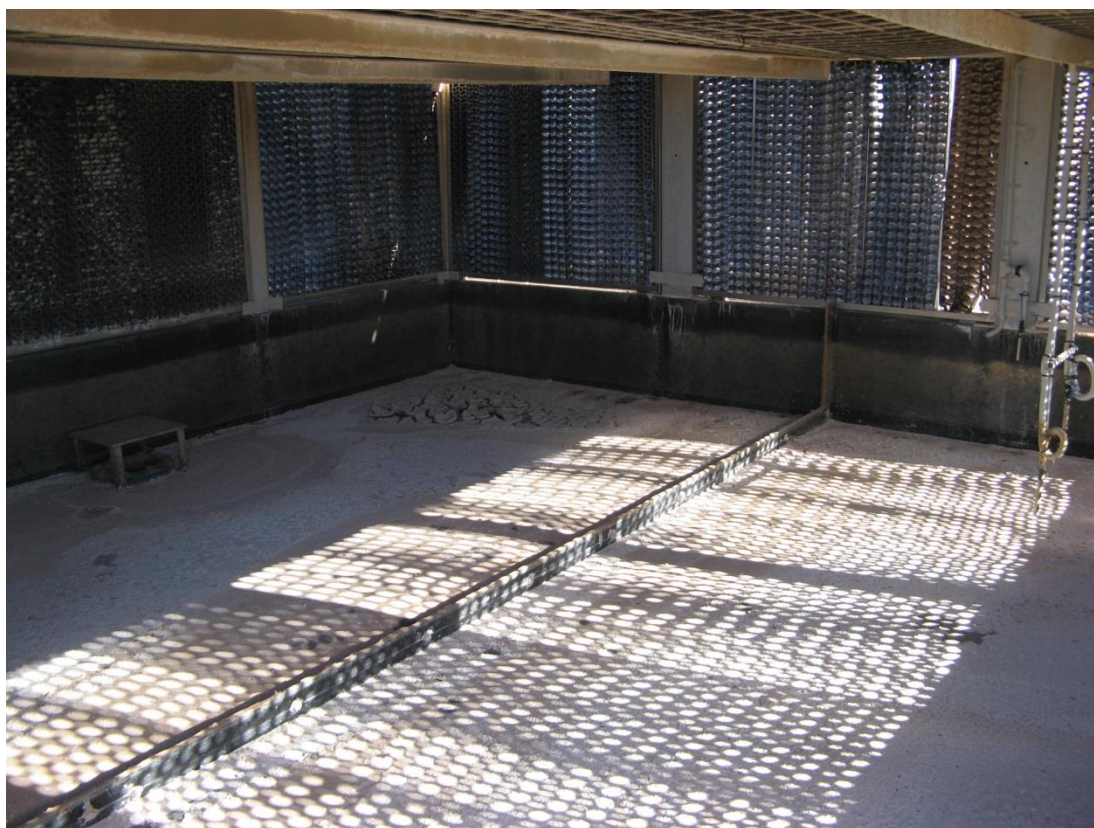
Figure 7.2. Mineral deposits developed at the base of one of the cooling towers at Thargomindah (Ryan, I 2014, supplied photograph, 25 March)
