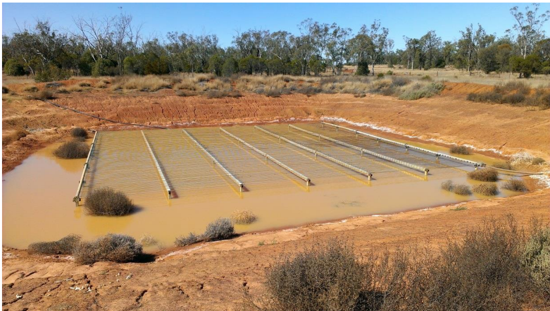
Figure 2.1. Submerged domestic copper pipe cooling grid at “Tabooba” (pond yet to be filled)
