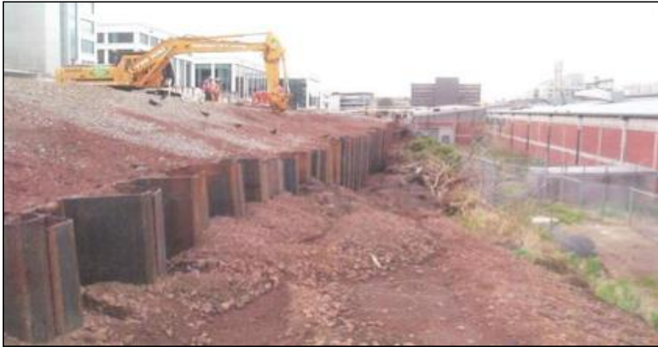
Figure 1-2: Cantilever Sheet Pile (Hauraki Pilling LTD)
