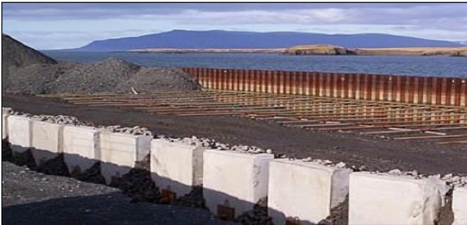
Figure 1-3: Macalloy Anchored Sheet Pile (Iceland, 2002)
