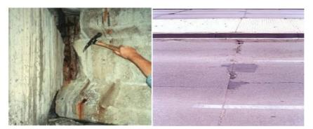
Figure 2.2 - ASR damaged structures (Fournier et all, 2010)
