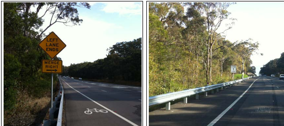
Figure 3.4 – Photographs of site 2 – Toronto Road
