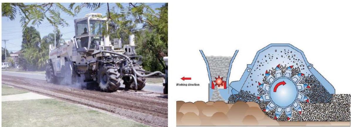
Figure 2-9: Direct injection spreading and mixing of lime (Ramanujam, Jones & Janosevic 2009)
