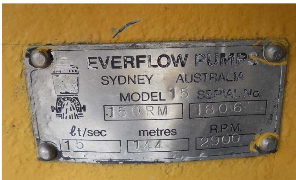
Figure 3.16: John Street bore pump label.
