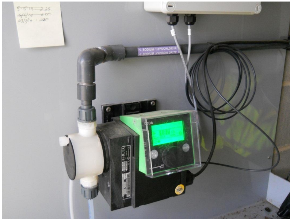
Figure 3.11: John St bore chlorination control unit.
