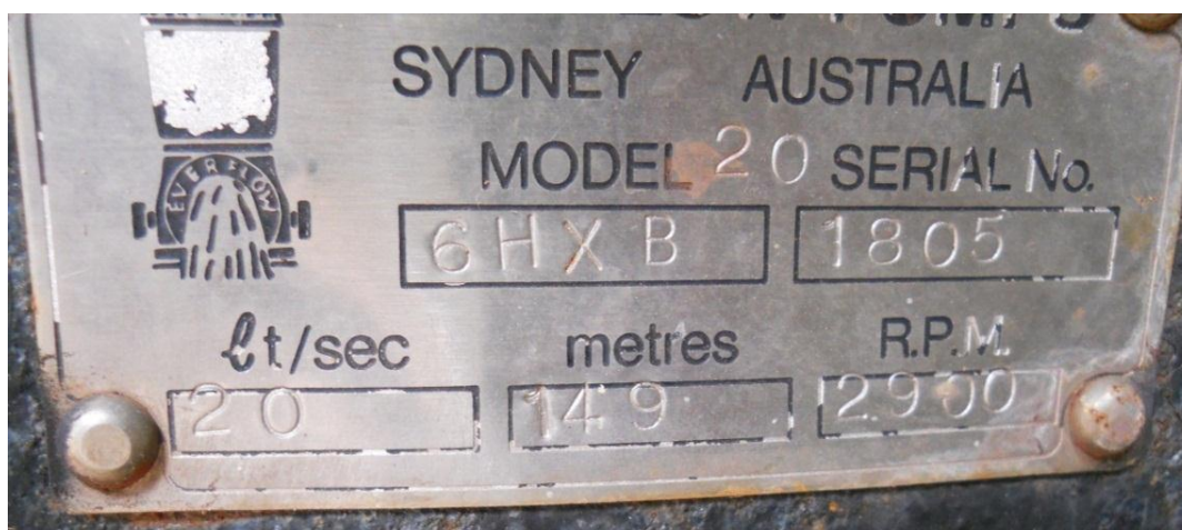
Figure 3.17: George Street bore pump label.
