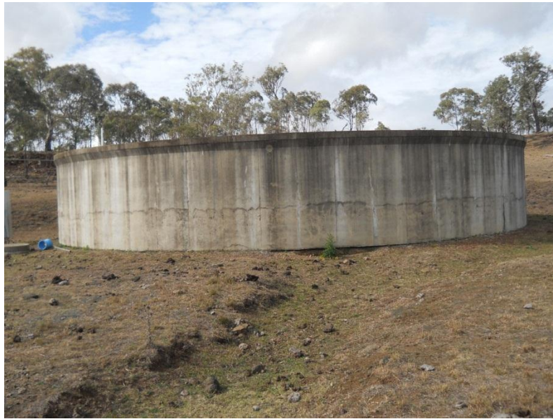
Figure 3.6: Cambooya's recently retired 400kL reservoir.
