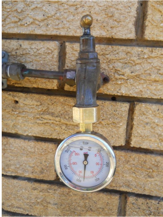
Figure 3.34: 28mm tap - Suited for pressure gauge connection.
