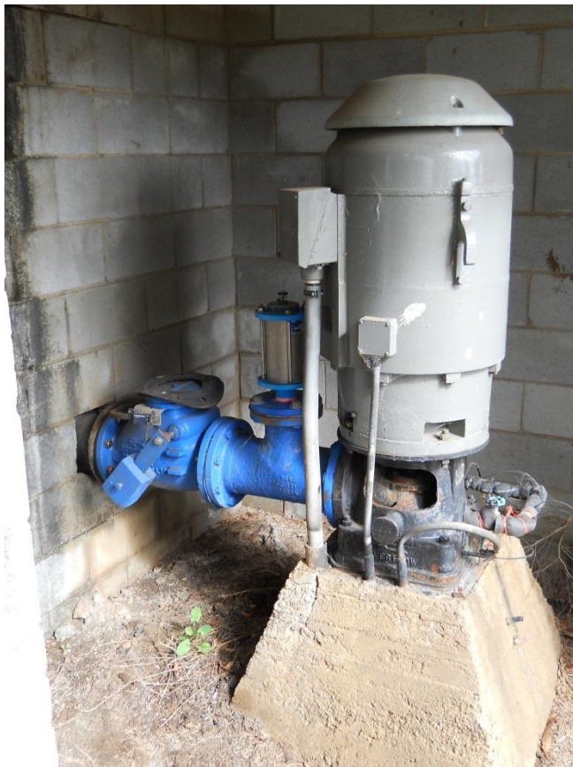
Figure 3.14: George St bore electric motor drive.
