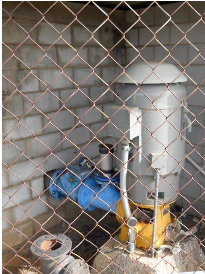
Figure 3.9: John St bore electric motor drive.
