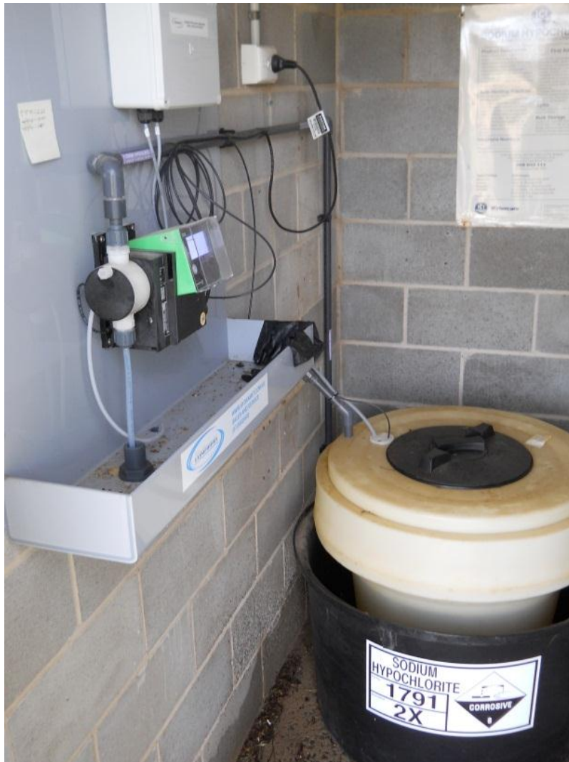
Figure 3.31: George St bore chlorination control unit & Sodium Hypochlorite basin.
