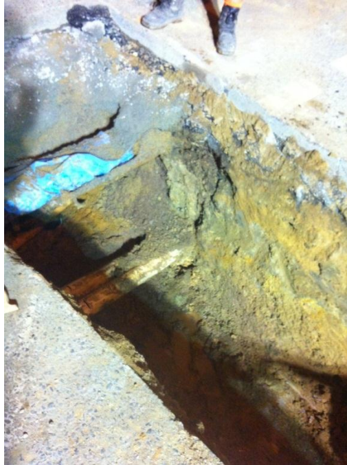
Figure 28: Service conflicts discovered during night works
