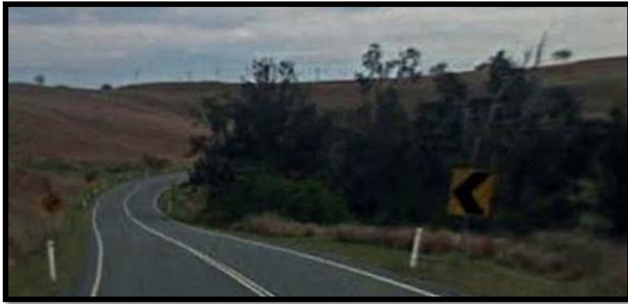
Figure 4- 9: Kooralbyn Road, Kooralbyn. Eight accidents on this road
