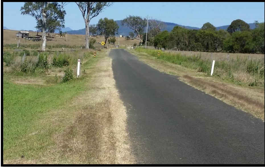
Figure 5- 10: Typical “Rural, undivided sealed, unsealed shoulders”. Allandale Road, Allandale
