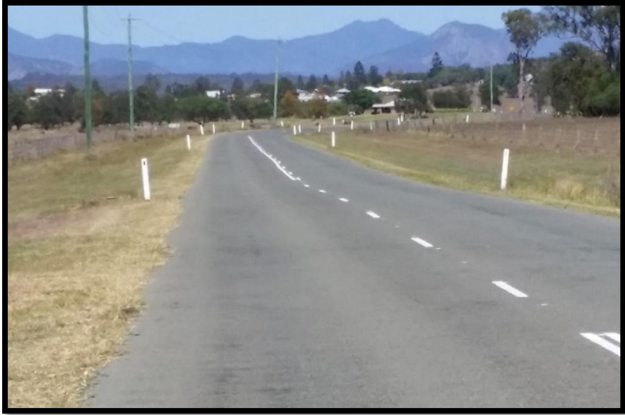
Figure 5- 9: Typical “Divided sealed, unsealed shoulders”. Allandale Road, Dugandan
