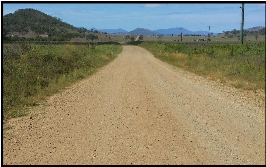
Figure 5- 11: Typical “Unsealed road”. Old Rifle Range Road, Coulson.
