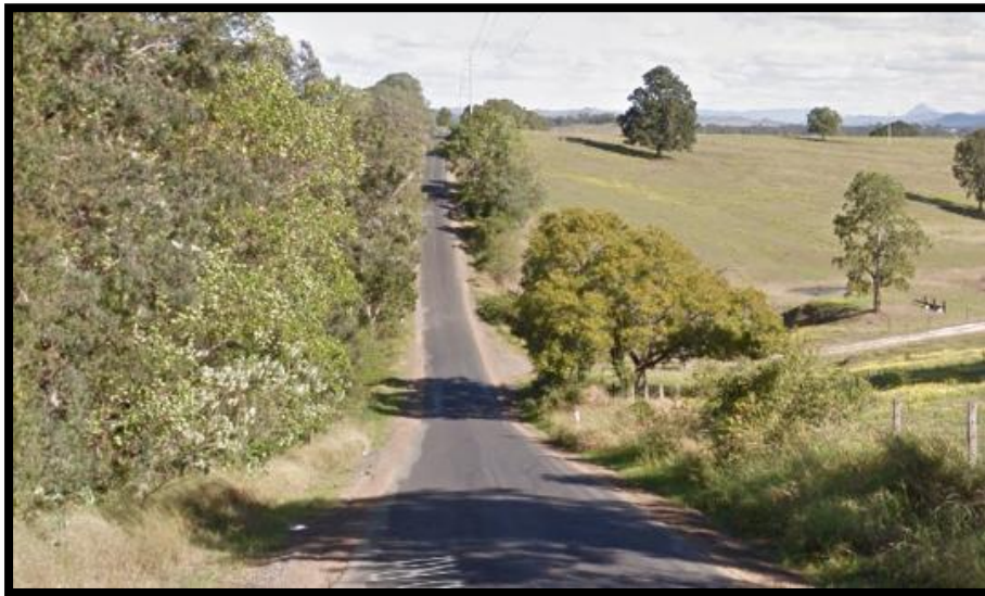
Figure 4- 10: Veresdale Scrub Road, Veresdale Scrub. Nine accidents including one fatality.
