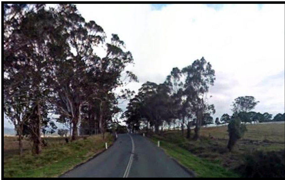
Figure 4- 8: Kerry Road, Kerry. Eight accidents including a fatality on this bend.
