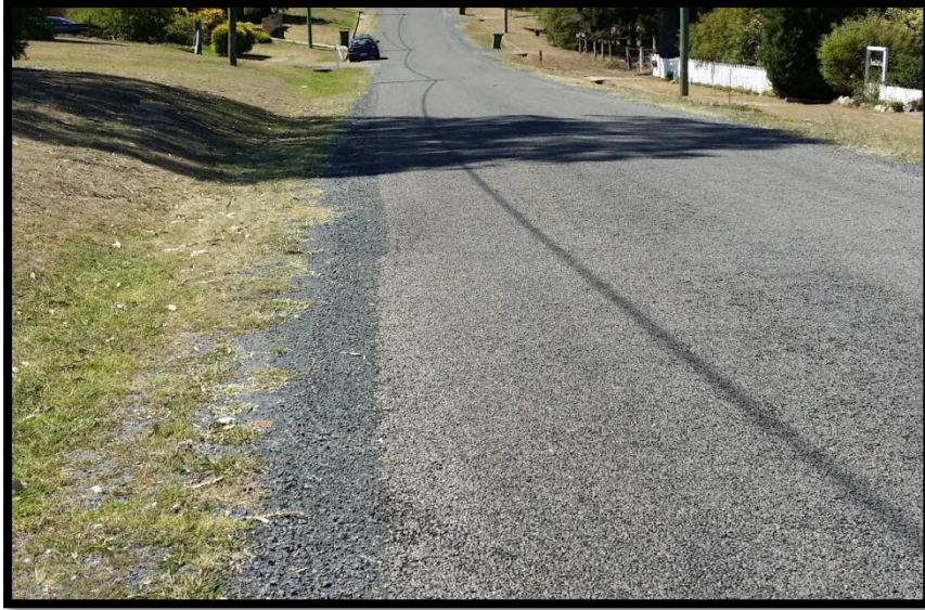
Figure 5- 8: Typical “Undivided sealed, unsealed shoulders”. Grace Street, Dugandan
