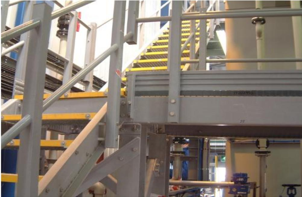
**Figure 4 Bolted connections on FRP staircase (Creative Pultrusions, Inc, 2008)**
