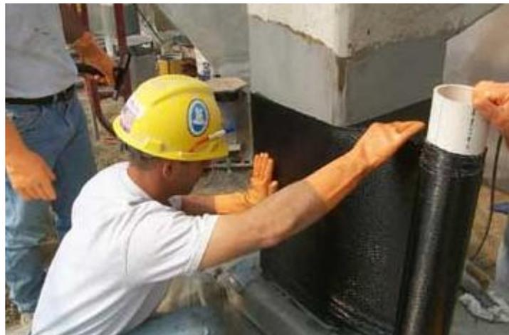
**Figure 2 Wrapping of column in FRP (Sika, 2012)**
