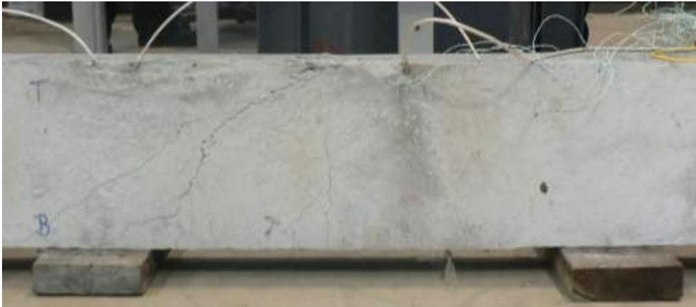
Figure 65 - Flexural and Shear Cracking of Control Beam
