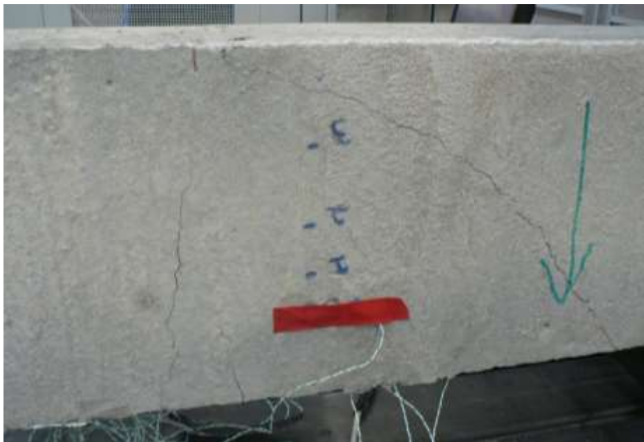
Figure 66 - Flexural and Shear Cracking of Heated Beam
