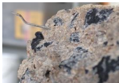
Figure 6.15: Steel fibre after flexural failure
