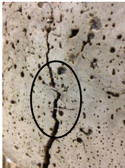
Figure 5.19: Crack bringing of Forta Ferro fibre
