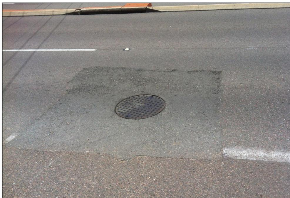
**Figure 2.1:** AC raised after asphalt overlay producing a poor surface, Bundock Street, North Ward.
