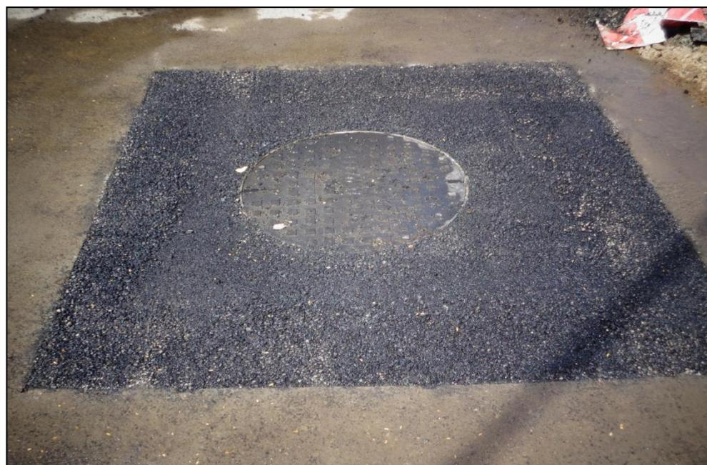
**Figure 2.8:** Reconstructed pavement around AC, China Street, Mundingburra.
