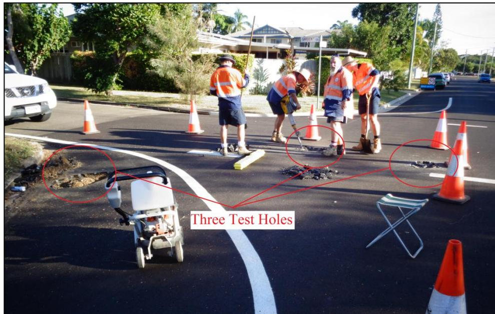
**Figure 2.4:** TCC crew locating the AC which was covered with asphalt, China Street, Mundingburra.
