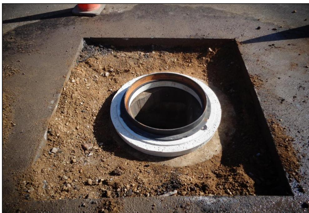
**Figure 2.6:** Concrete riser ring and circular cast iron AC frame installed, China Street, Mundingburra.
