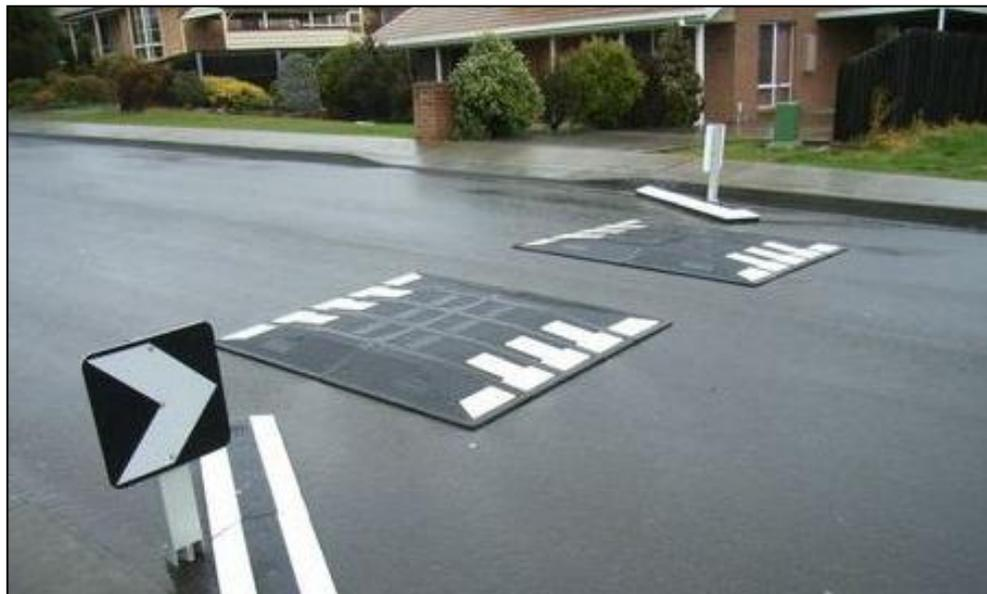
**Figure 1.3:** Recycled rubber speed cushion and kerb (Saferoads Pty Ltd, 2011).
