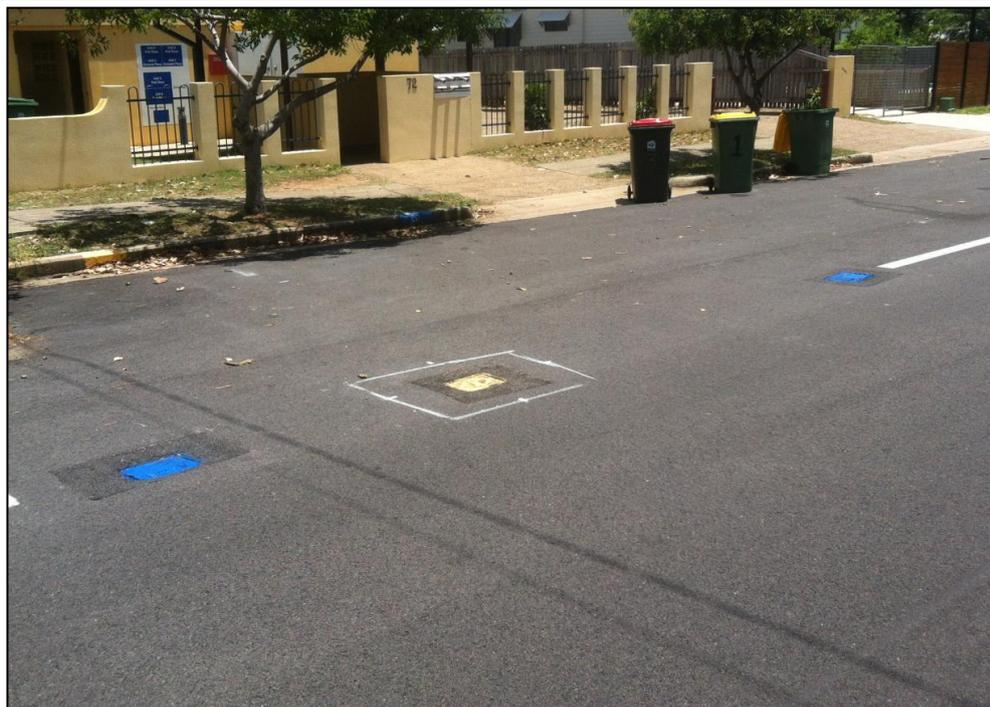
**Figure 2.2:** Valve boxes raised after overlay producing a poor surface, Stagpole Street, West End.
