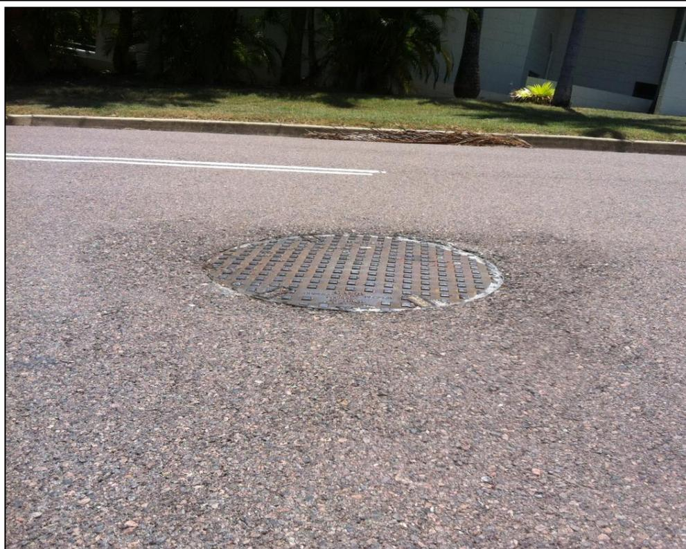
**Figure 2.3:** Asphalt ramped to AC resulting in a 30.0 mm depression, Little Street, North Ward.
