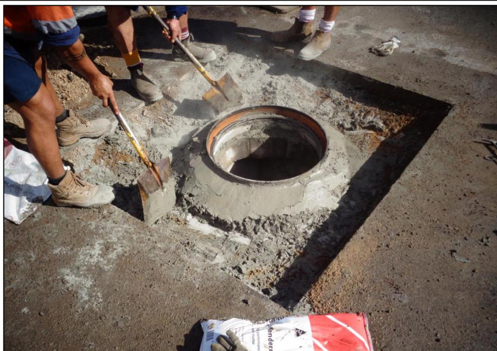
**Figure 2.7:** Grouting and sealing AC frame to the concrete slabtop, China Street, Mundingburra.
