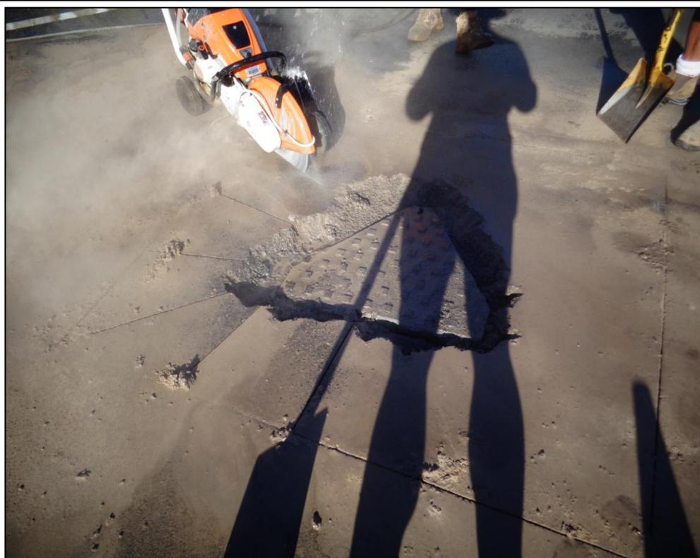
**Figure 2.5:** TCC crew cutting around the AC creating a square patch, China Street, Mundingburra.
