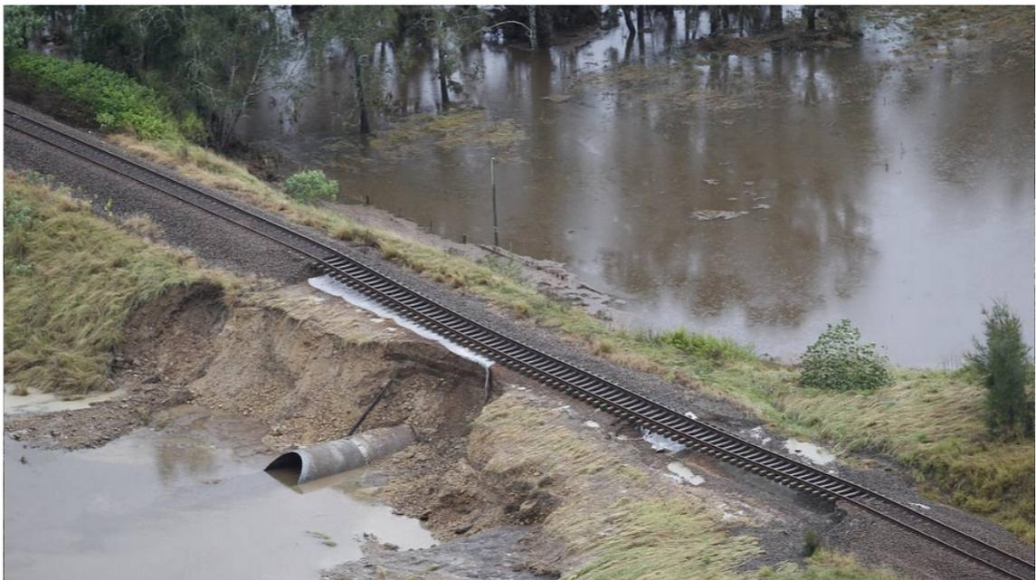
Figure 38: Damaged rail culvert - Newcastle 2015 flood (Source The Herald, 2015)
