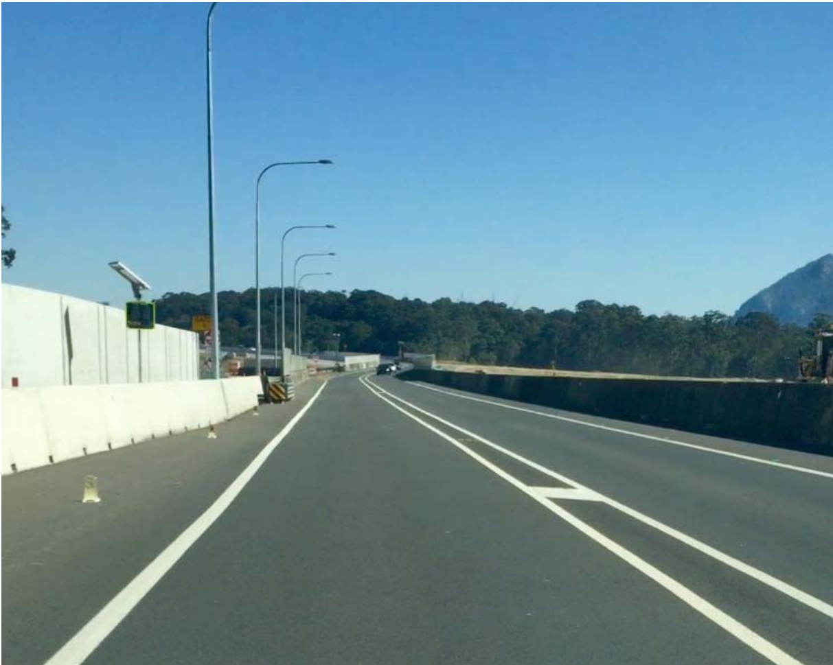
Figure 5.1: Data Collection Site: Bruce Highway Upgrade – Cooroy to Curra, Pomona QLD – Perspective view
