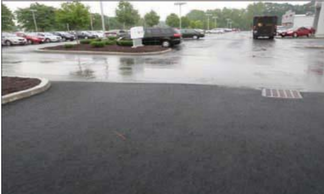
Figure 8: A picture depicting the differences between Permeable Concrete and traditional asphalt. Note the obvious differences between the foreground and background that represents the accumulation of stormwater runoff and pollution on traditional concrete. (Lake George Association, 2012).
