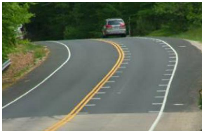
Figure 2 Optical Speed Bars (McGee and Hanscom, 2006)
