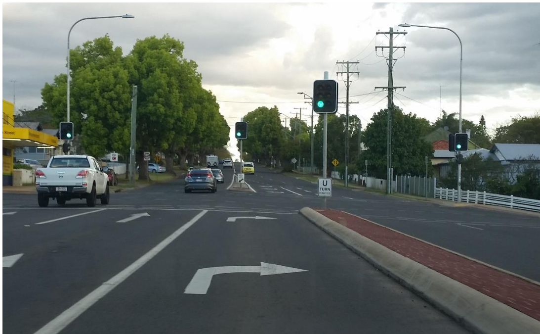
Figure 1 - Photo of Right Turn Filter Traffic Signal
