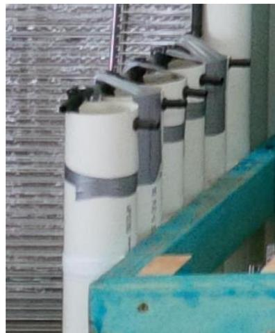
*Figure 4.6: Fitted nozzles installed in bored drainage holes*
