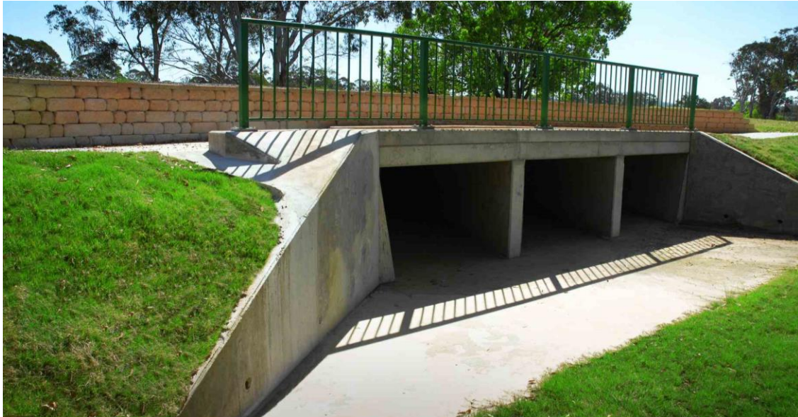
Figure 5: New England Highway Stormwater Culvert (Kehoe Myers 2015a)
