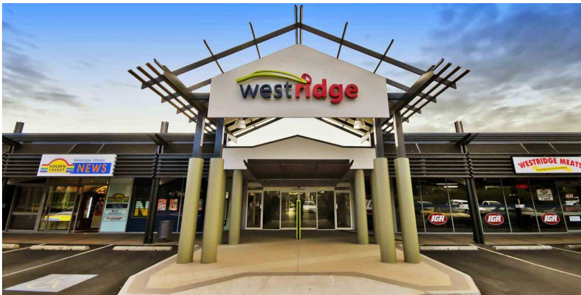
Figure 2: Westridge Shopping Centre (Kehoe Myers 2015a)
