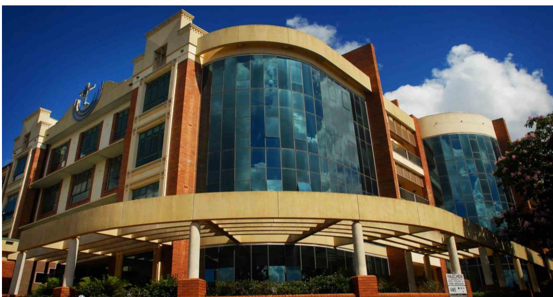
Figure 4: St Vincents Hospital (Kehoe Myers 2015a)
