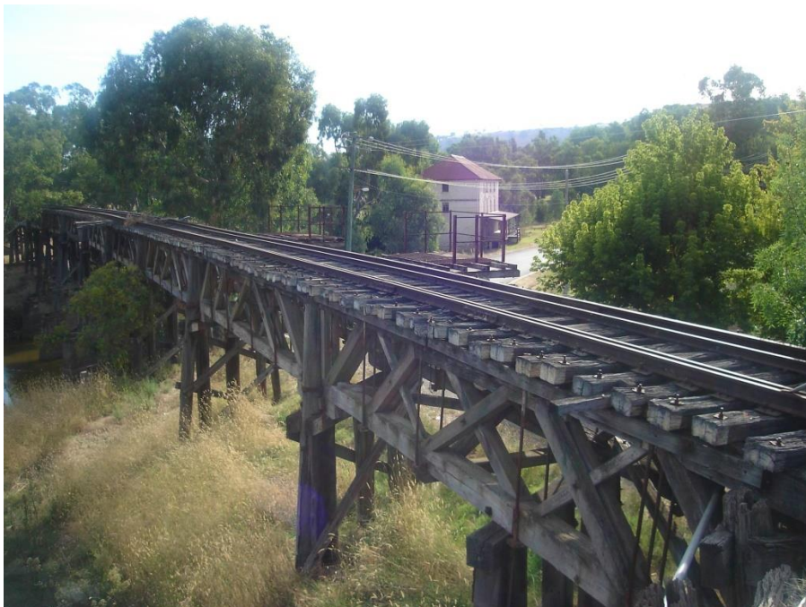
Figure 1: Open Deck Bridge (Yong, 2009)
