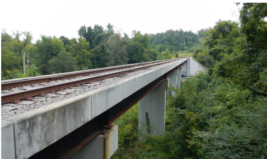
Figure 2: Ballast Deck (Crouch Engineering, 2014)
