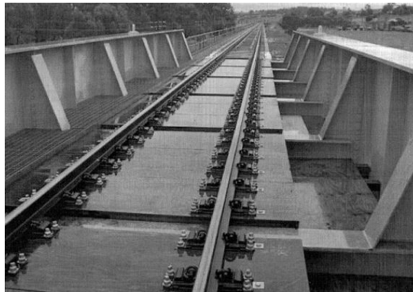
Figure 4: Example Transom Decking
