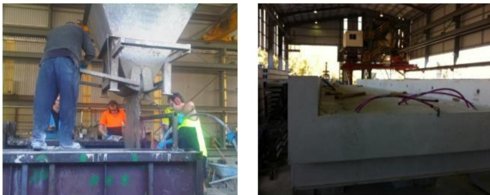
Figure 1-1 Production of Precast Concrete Products (Glasby 2012)
