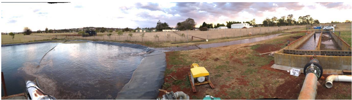
Figure 4.15 Panoramic view of water flowing from dam into flume and returning to dam
