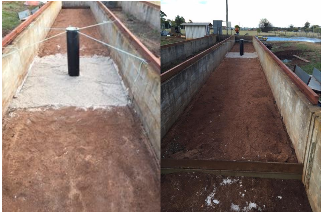
Figure 4.13 Flume showing control pier in positon, sand filled and slot for boards to water control depth
