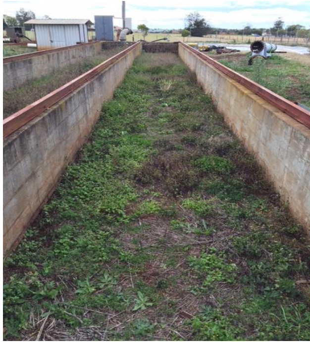
Figure 4.1 Large Flume at University of Southern Queensland
