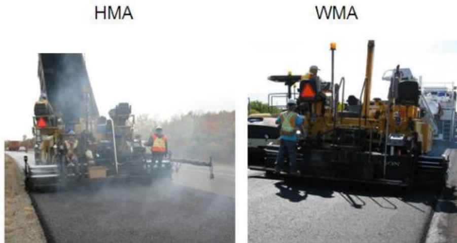
Figure 6: Comparison of Hot mix asphalt and warm mix asphalt (Politano, L 2012).
