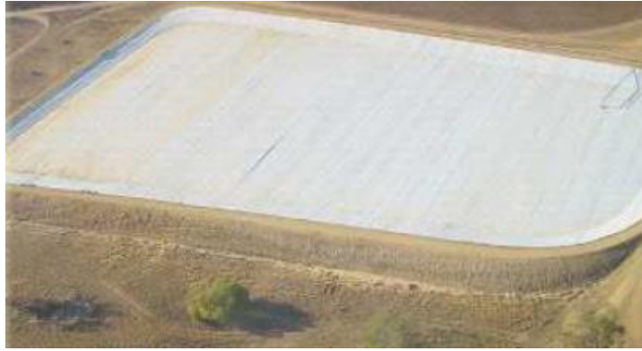
Figure 2.2: Continuous floating covers in use at St George, QLD (Craig, 2008)
