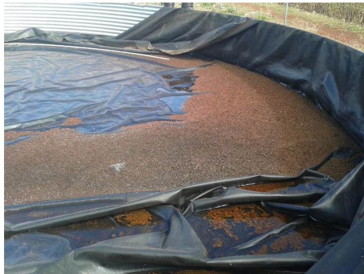
Stagnate water pooled on plastic liner
