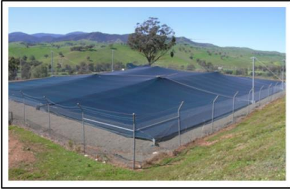
Figure 2.7: SuperSpan suspended impermeable covers (Finn & Barnes, 2007)
