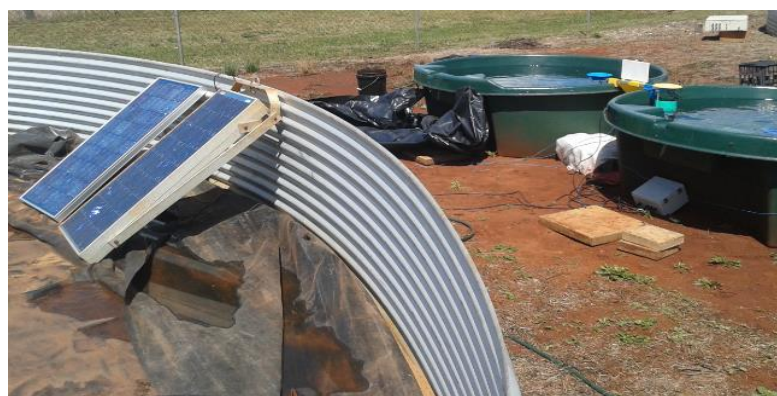
Figure 3.4 Solar panels (250watts)
