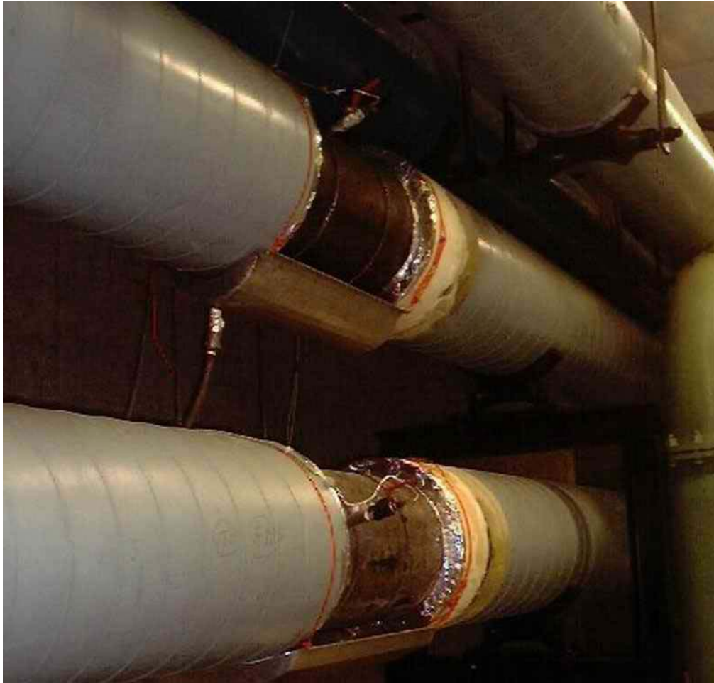
Figure 5.2: Installation of the Thermometers
