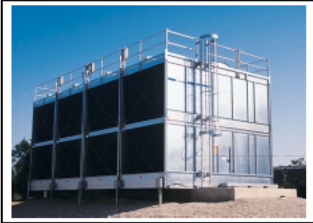
Figure 2.3: Typical Induced Draft Cooling Tower
