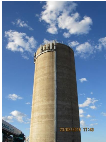
Figure 17: Communications facility mounted to a grain silo (Adams 2016)
