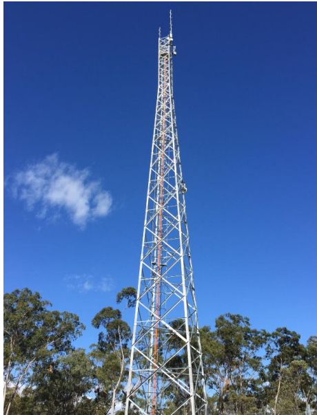
Figure 15: Self-supporting Tower (Adams 2016)
