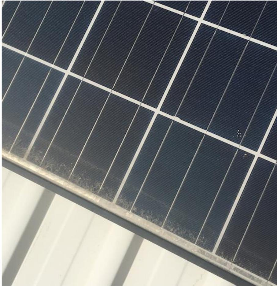
Figure 4.7 - Ingress and dirt on panel before cleaning causing heating.
