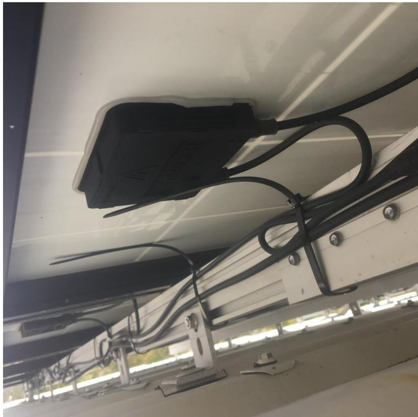
Figure 4.20 - Junction box located between 2<sup>nd</sup> and 3<sup>rd</sup> cell on 1<sup>st</sup> row.
