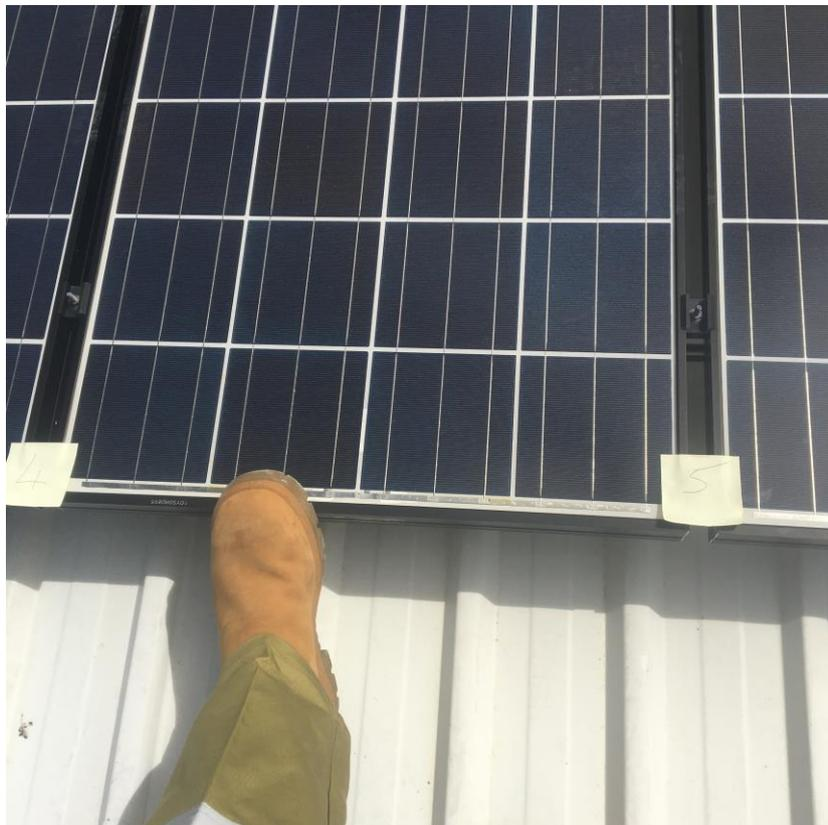
Figure 4.22 - 2<sup>nd</sup> picture taken of yellow post-it note showing panel 4 and foot indicating hot cell from figure 4.21.
