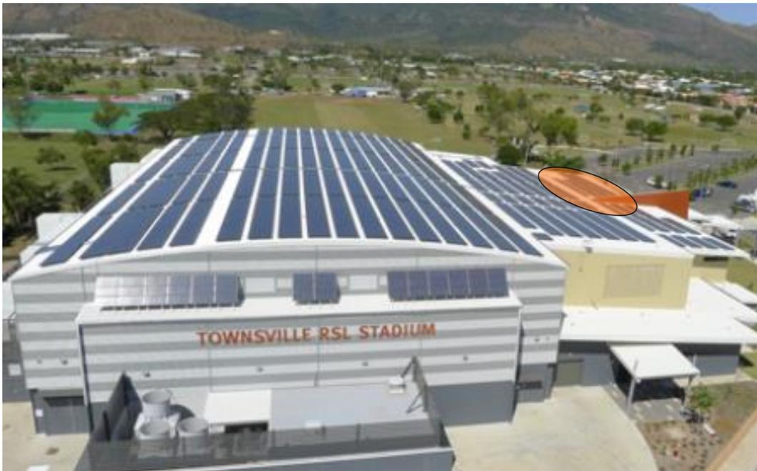
Figure 3.13 - RSL Stadium Solar Farm, scanned area in orange (Kyocera, 2012).
