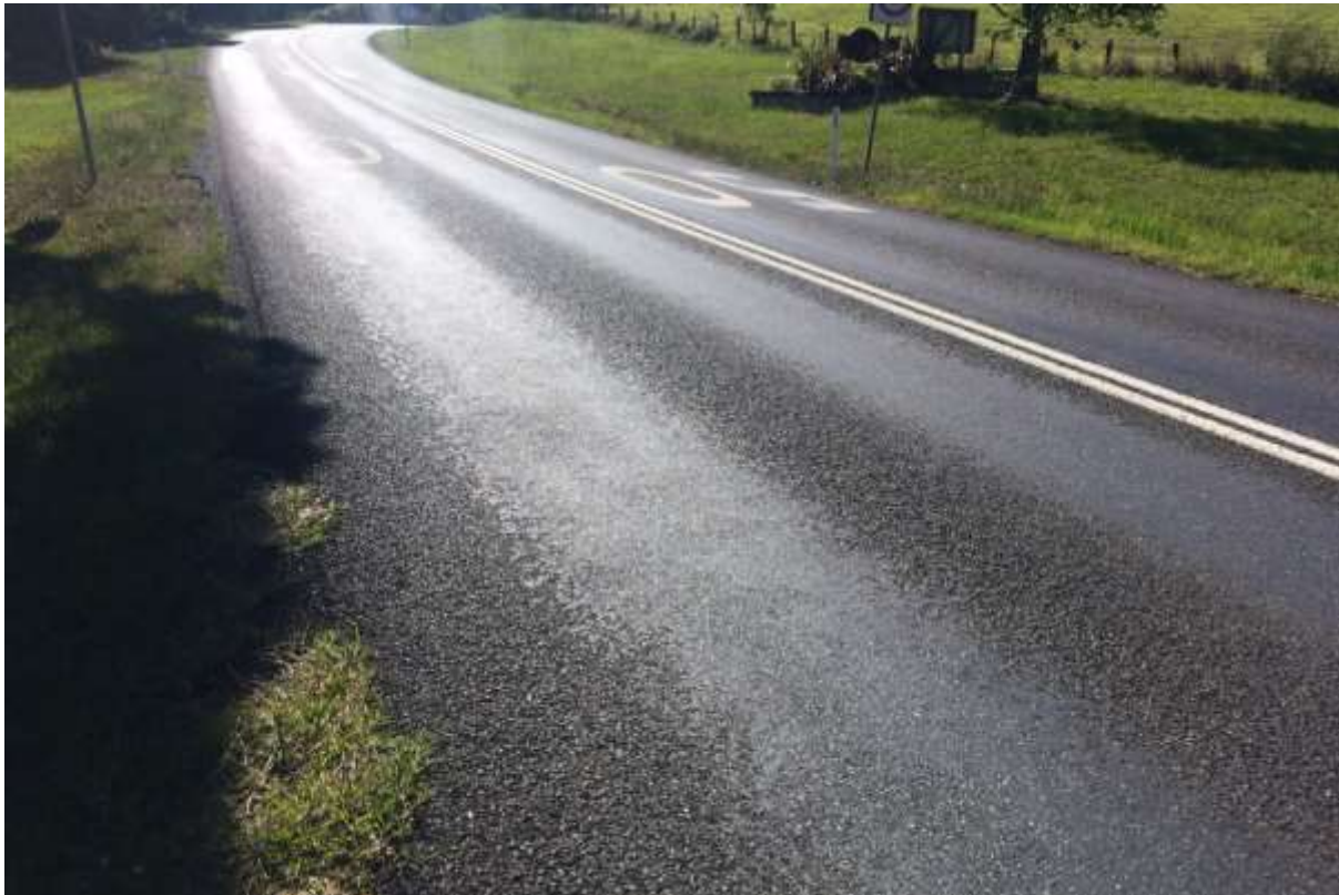
Figure 2.9: Example of flushing on local road with rutting also visible in the right lane.
