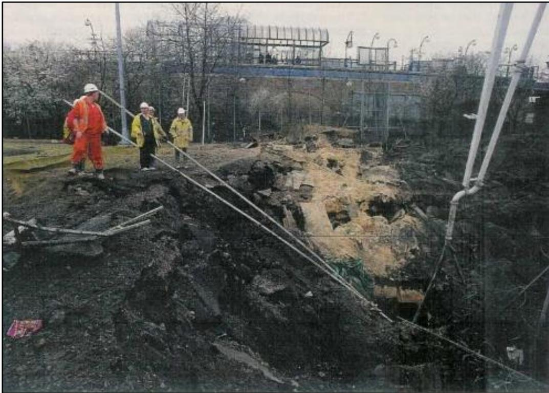
Figure 5.4: Sinkhole caused by blowout (Institution of Civil Engineers 1998).
