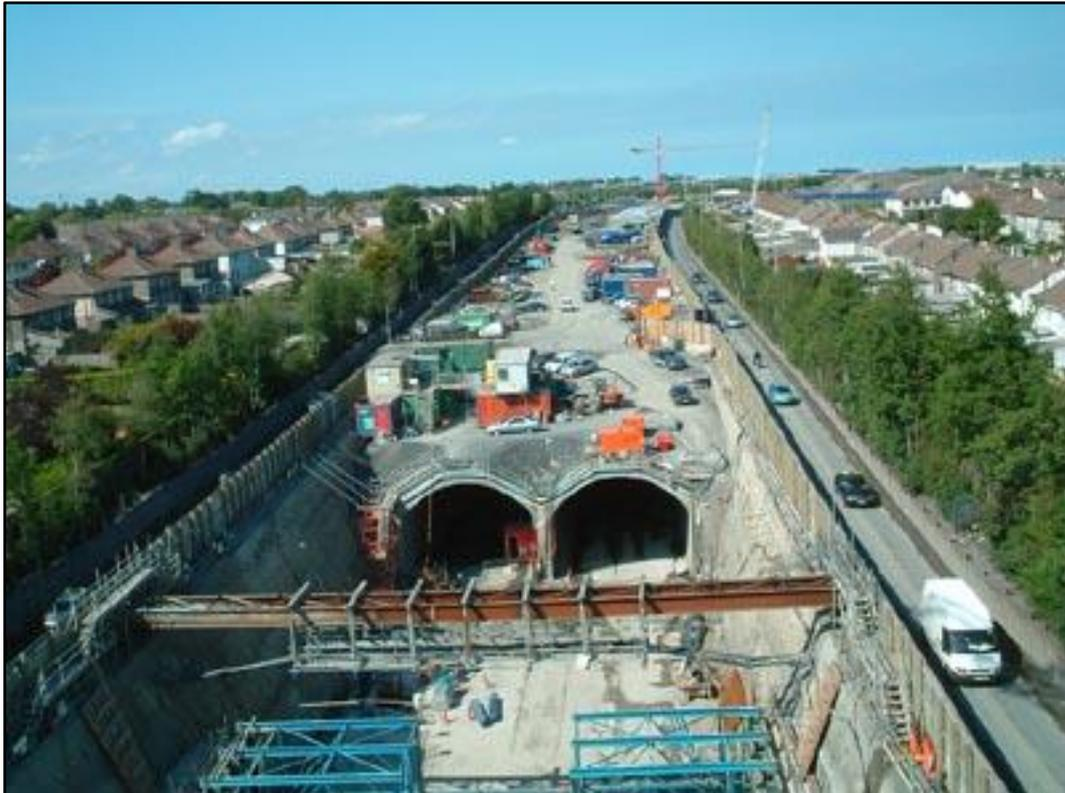
*Figure 2.7: Example of bottom-up cut and cover tunnelling (Wallis 2002).*
