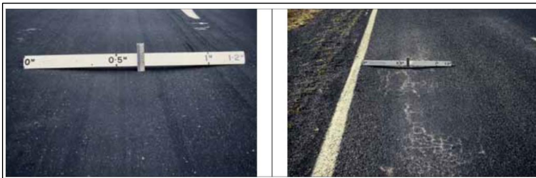
Figure 8 Typical Rutting
