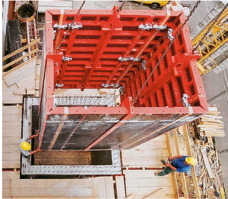
Figure 2-13 Peri Modular Panel Wall Formwork (Peri, 2016)
