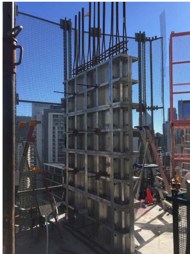
Figure 2-14 Aluminium modular panel form onsite at Abian Towers Brisbane
