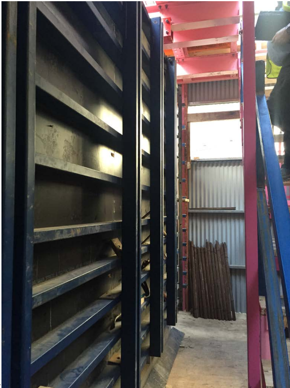
Figure 3-3 Steel Frame RHS Wall Forms within Jump Form at 300 George St Brisbane
