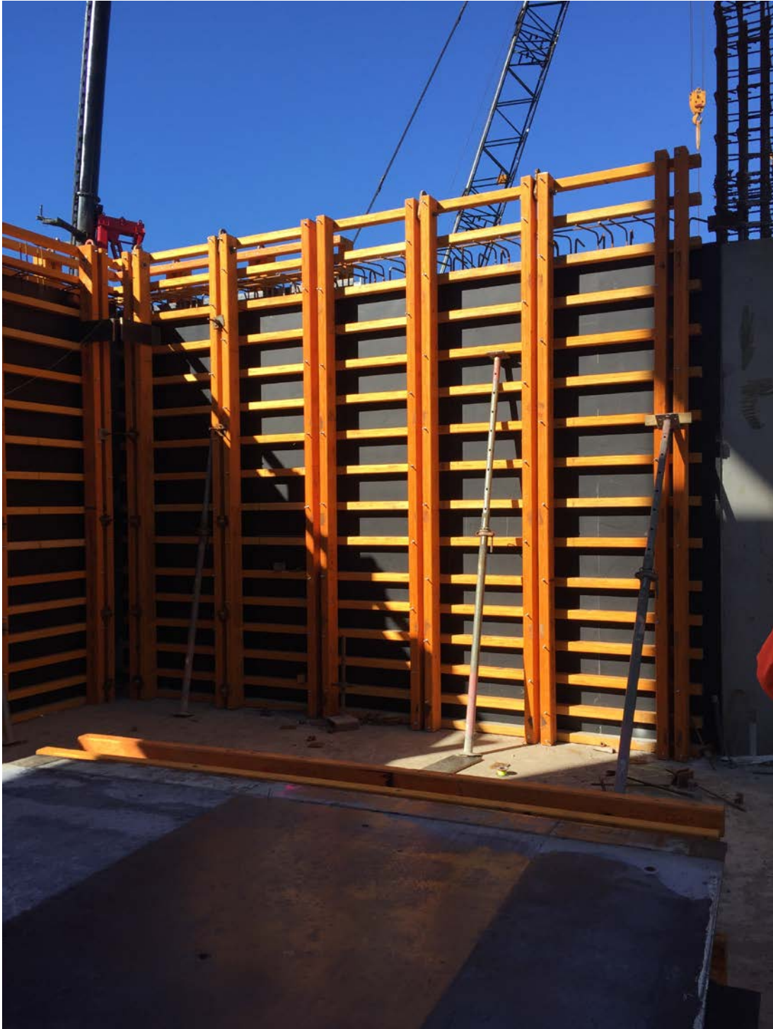
Figure 3-4 Timber LVL Wall Forms onsite 300 George St Brisbane
