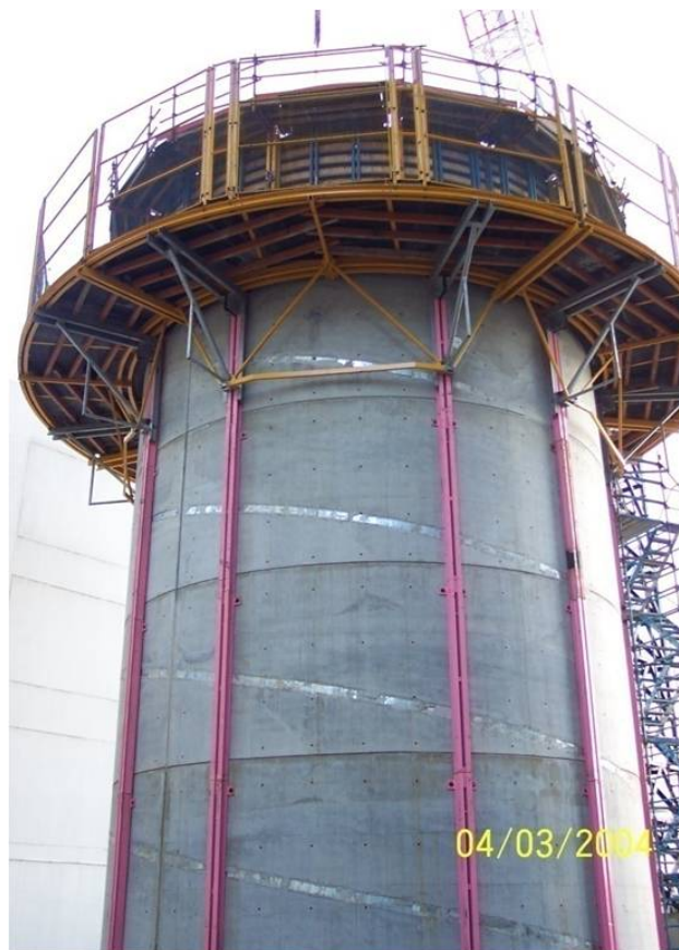
Figure 2-3 Crane Lifted Forming Platform System
