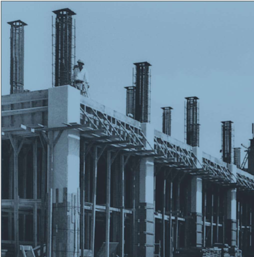
Figure 2-16 Stay in Place Forms – Precast Concrete Panels serving as Column Forms (ACI, 2005)
