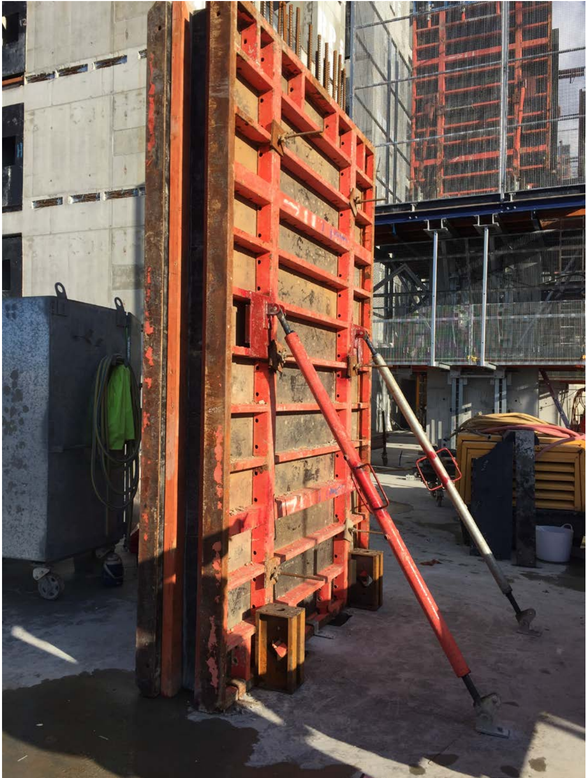
Figure 2-15 Manufactured Modular Panel Forms onsite at 320 Hay St Perth
