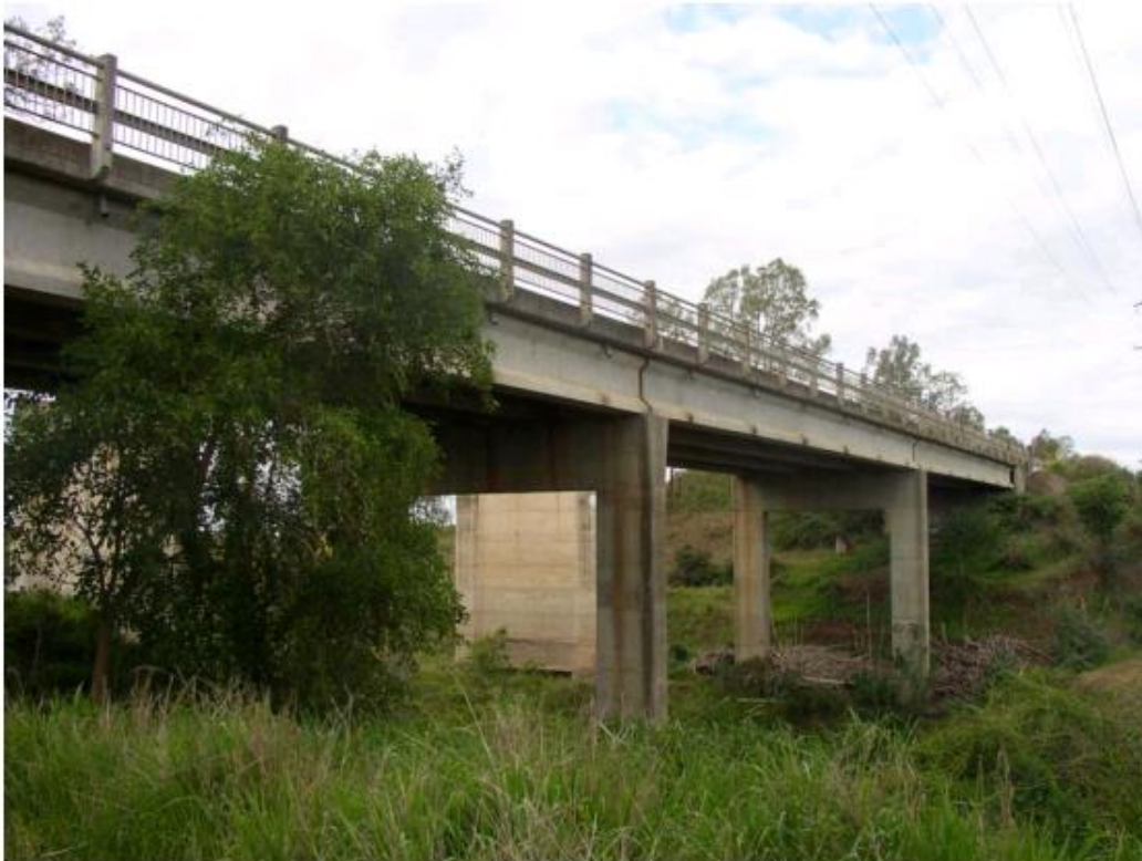
Figure 4.1, Tenthill Creek Bridge (Setunge 2002)
