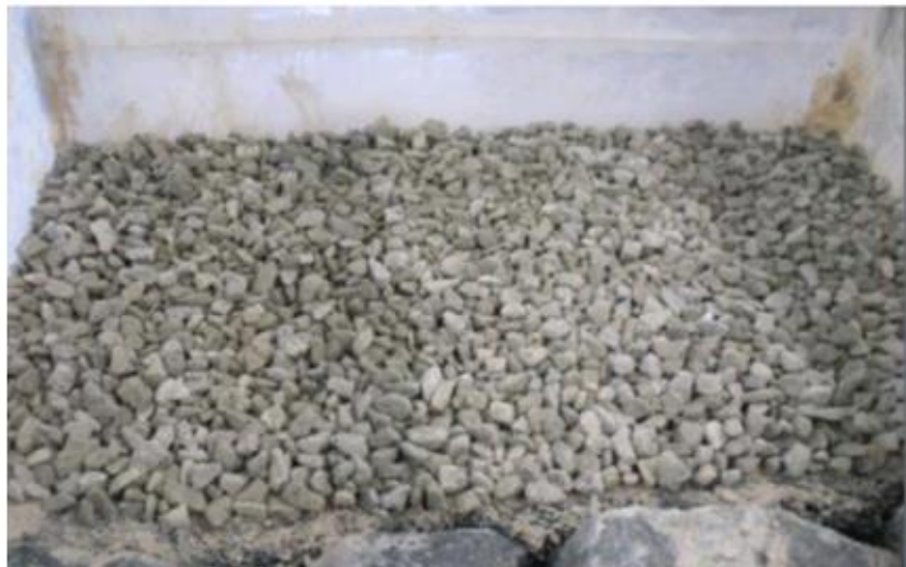
Figure 3.18, Gravel underlayer on the levee (Johnson et al., 2013)
