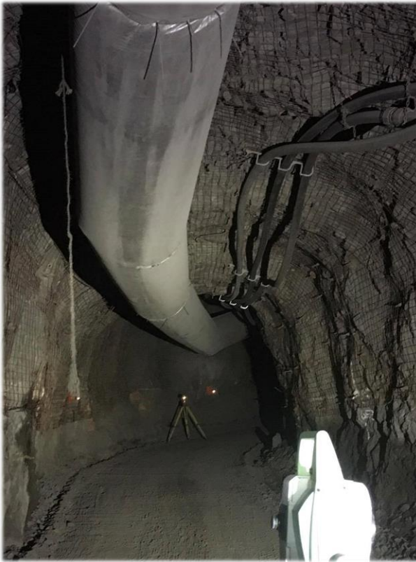
Figure 3-3 Check Survey traversing up the Incline
