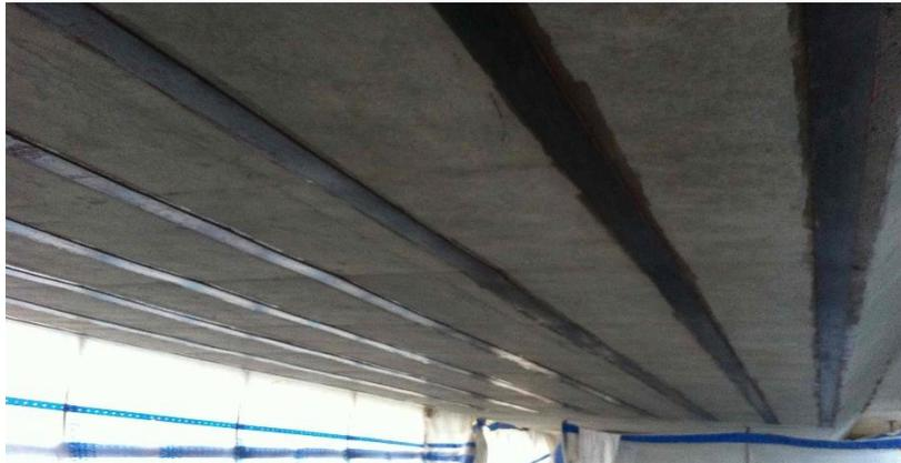
**Figure 2-1 Surface Mounted CFRP Reinforcing, Caswell Drive, Canberra**
