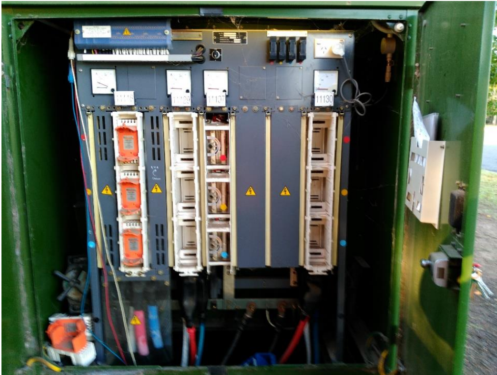
Figure 6: LV board of Tx with manual data logger connected
