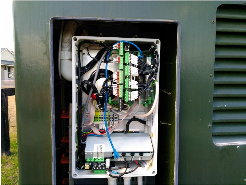
Figure 20: Interior of a DM&C unit installed on a distribution Tx
