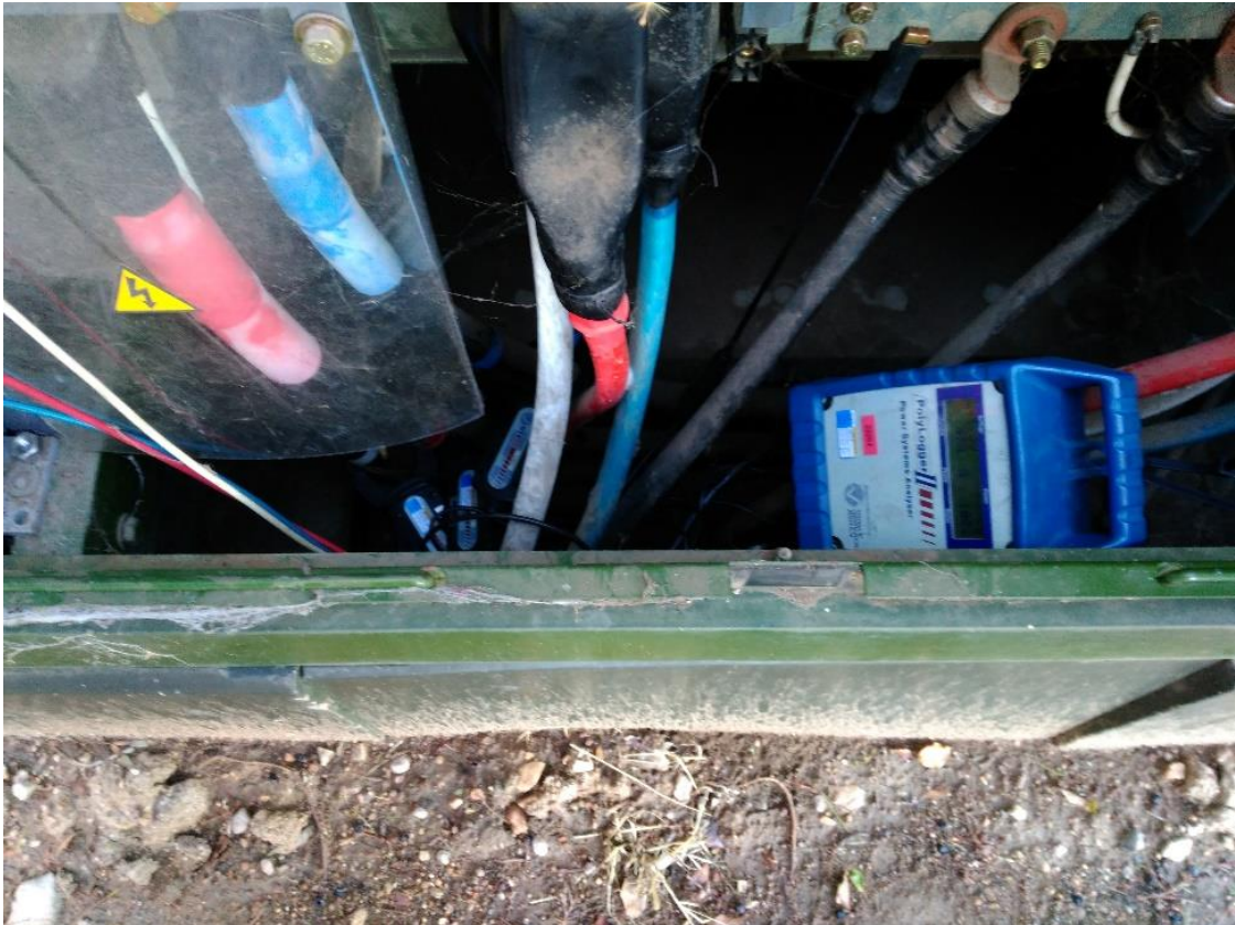
Figure 49: Direct distributor showing CT's and data logger installed
