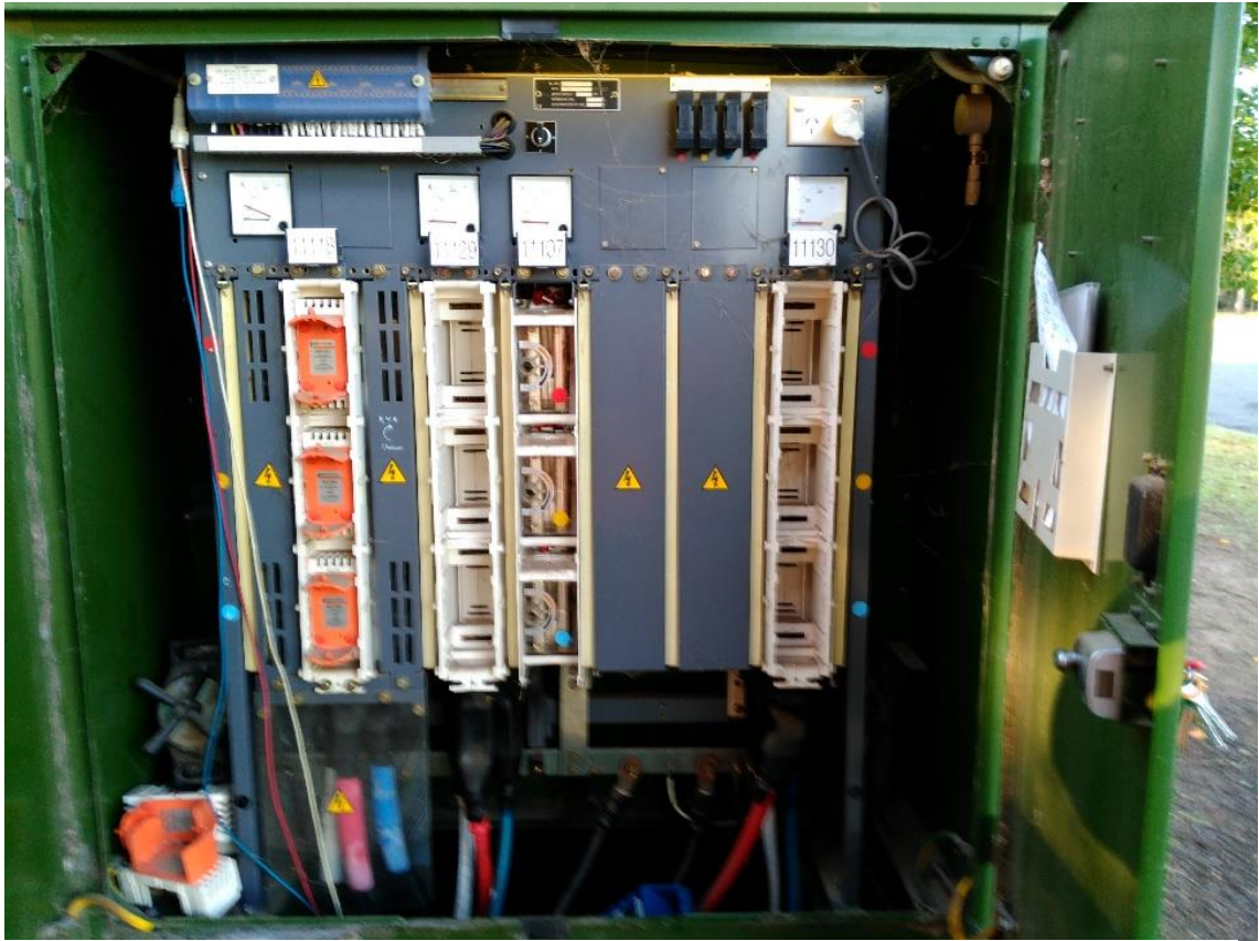
Figure 48:: Kiosk LV board showing data logger voltage leads installed
