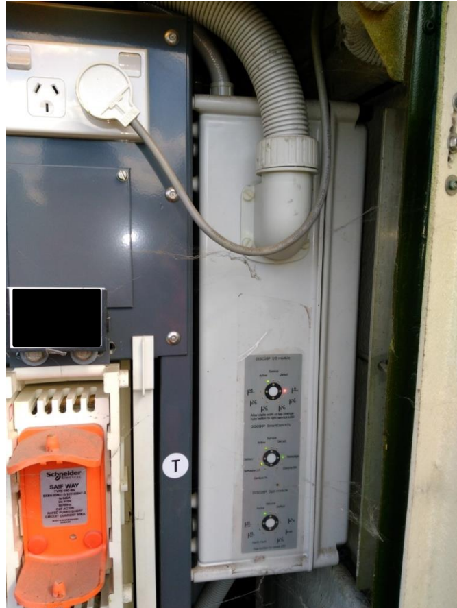
Figure 19: Exterior of DM&C unit installed on a distribution Tx
