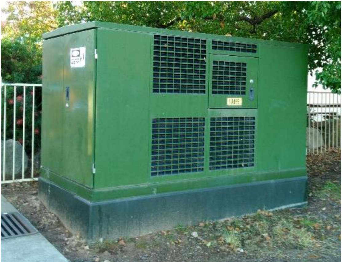
Figure 47: Kiosk Transformer
